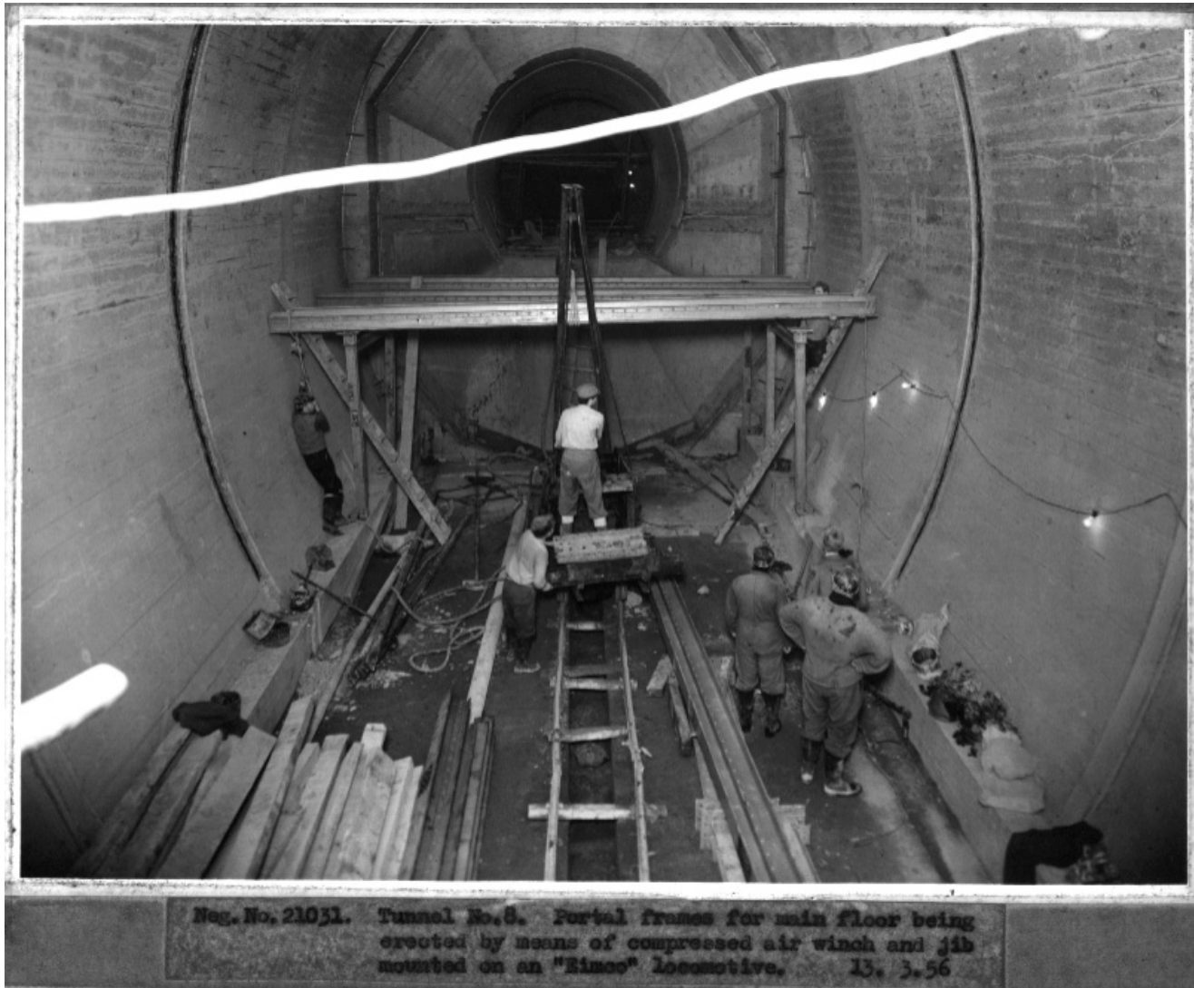
ABOVE. Fig.4.009. Original photography documenting the construction of the GUTE, March 1956. The scale of the main tunnel is evident and this was subdivided to create two working levels. [Source: Photograph by tunnel engineer Patrick Gough. Courtesy of George Coney]
