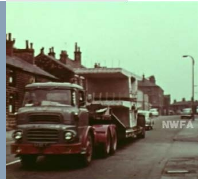
ABOVE. Fig.2.030. Pre-cast units transported to site by lorry [Source: Mancunian Way, 1967. Author's screen grab. Courtesy North West Film Archive & Concrete Society]
