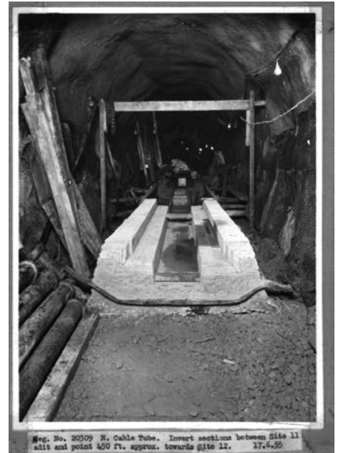
ABOVE. Fig.4.010. Original photography documenting the construction of the GUTE, June 1955. Work in progress on one of the long cable tunnels. [Source: Photograph by tunnel engineer Patrick Gough. Courtesy of George Coney]
