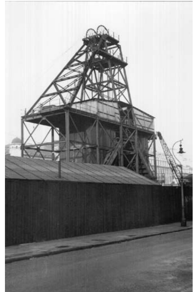
ABOVE. Fig.4.015. Prominent headgear, located in Piccadilly, needed to winch man and materials up and down the shaft to the GUTE tunnel workings. [Source: Photograph by tunnel engineer Patrick Gough. Courtesy of George Coney]
