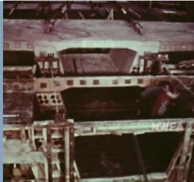
ABOVE. Fig.2.029. Pre-casting of road sections at Len Fairclough's casting yard in Adlington, near Chorley [Source: Mancunian Way, 1967. Author's screen grab. Courtesy North West Film Archive & Concrete Society]
