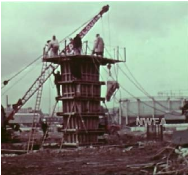
ABOVE. Fig.2.028. In-situ casting of columns [Source: Mancunian Way, 1967. Author's screen grab. Courtesy North West Film Archive & Concrete Society]
