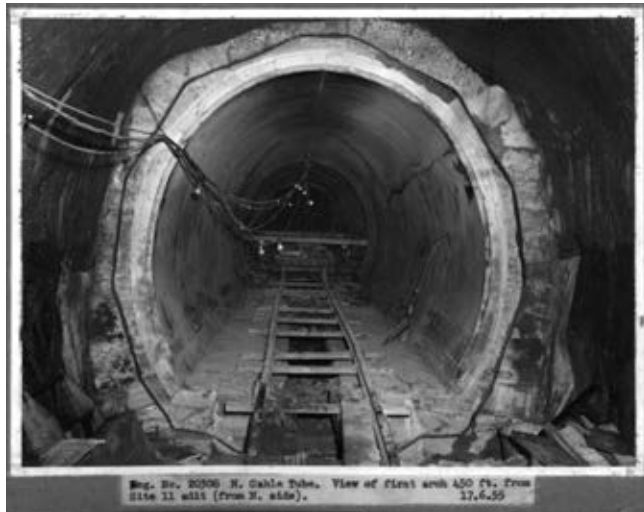
ABOVE. Fig.4.011. Original photography documenting the construction of the GUTE, June 1955. Another view of work in progress on the cable tunnels. [Source: Photograph by tunnel engineer Patrick Gough. Courtesy of George Coney]
