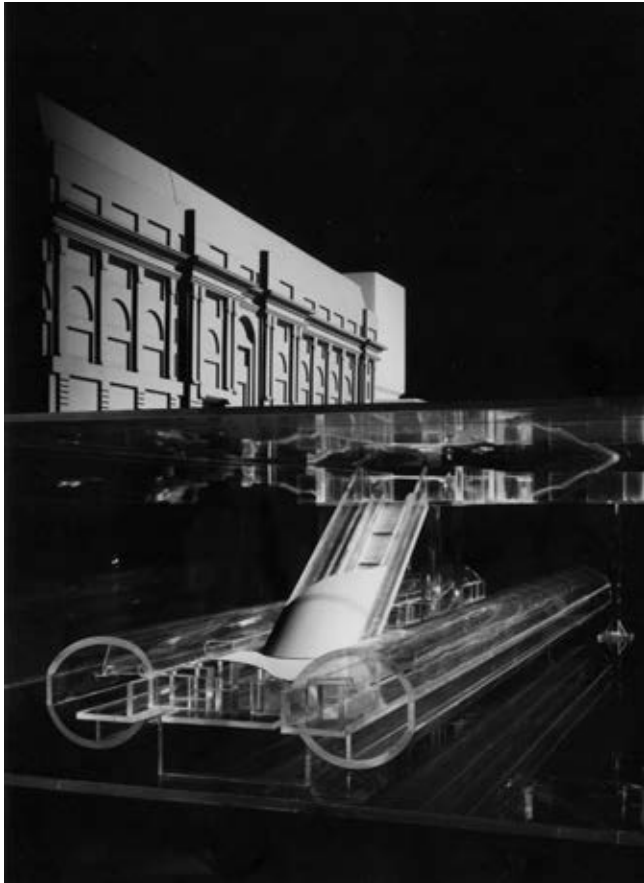
ABOVE. Fig.3.040. Perspex model of Royal Exchange station as proposed with existing exchnage building in a solid material [Source: Museum of Transport Greater Manchester. Uncatalogued photos held in SELNEC archive. Author's scans]
