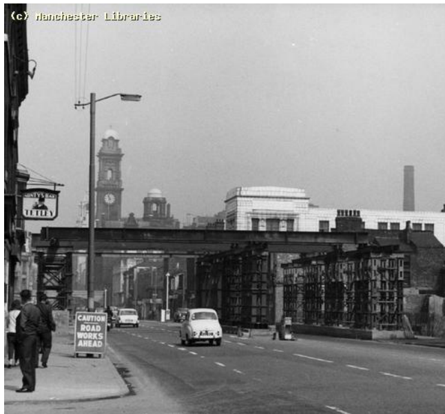
ABOVE. Fig.2.031. Preparations for the in-situ casting of the central section over Oxford Road [Source: Johnstone, W.M. 1960 Oxford Road, Building of Mancunian Way, M03830. Manchester Libraries Local Image Collection. Manchester Central Library, Local Studies Unit]
