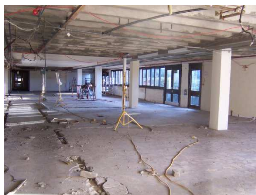
Figure 3. The Special Collections building in construction
