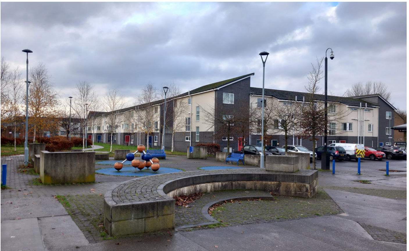
Top: The First House Community Hub in Brinnington. Bottom: Part of the public plaza outside First House
