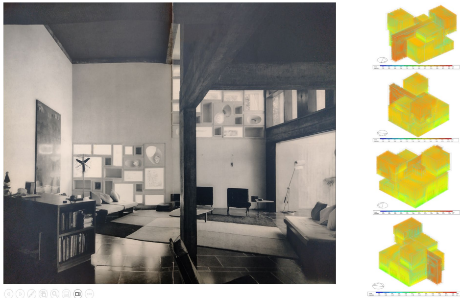
Figure 10. Interior photograph of the Shodhan house showing the latticed shaded openings from inside, the double height voids, the ferroconcrete frame and the standing fan. 19
