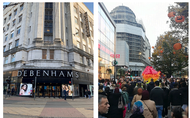
Fig. 5. Debenhams department store opened (left: 13 February 2019. Source: http://www.moneybright.co.uk/ ) and its ruins during Monsters Rock! Party Procession on Market Street (right: 29 October 2023, 3:56 PM. Source: Author 1).
