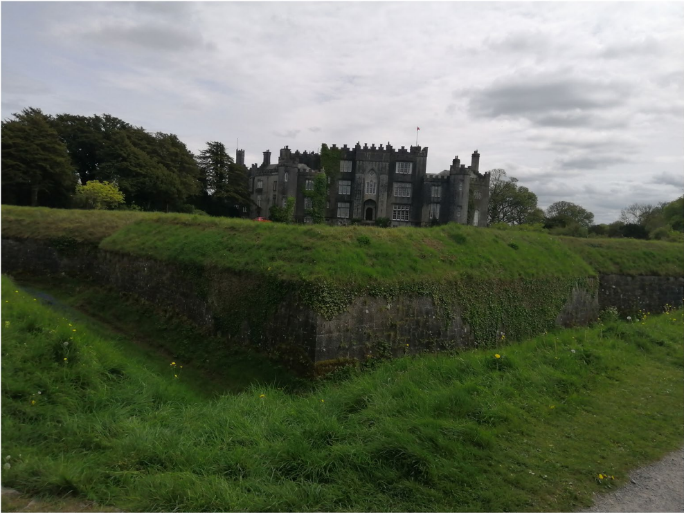
Figure 1. View directly facing the bastion and castle. The use of ramparts elevates the opposite side of the ditch, though have lost definition over the years. Source: produced by author.
