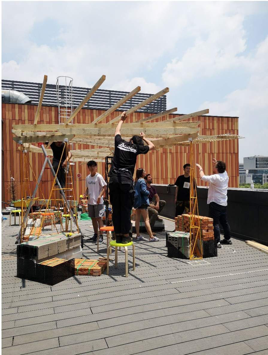
Figure 3. Construction process. Source: Sofia Quiroga 2018*
