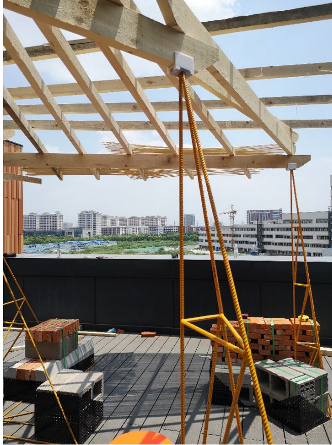
Figure 4. Construction process. Source: Sofia Quiroga 2018*
