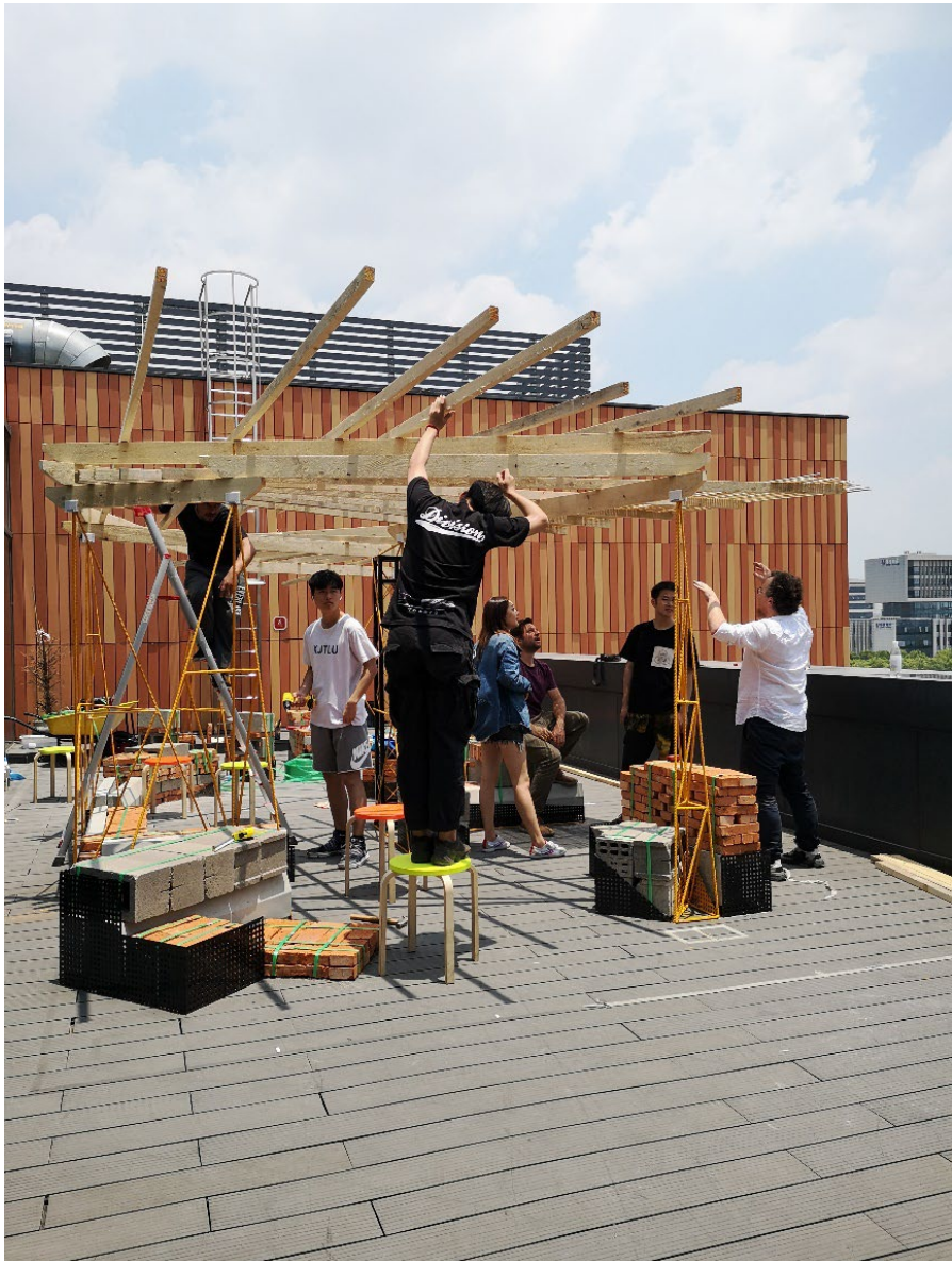
Figure 3. Construction process. Source: Sofia Quiroga 2018*
