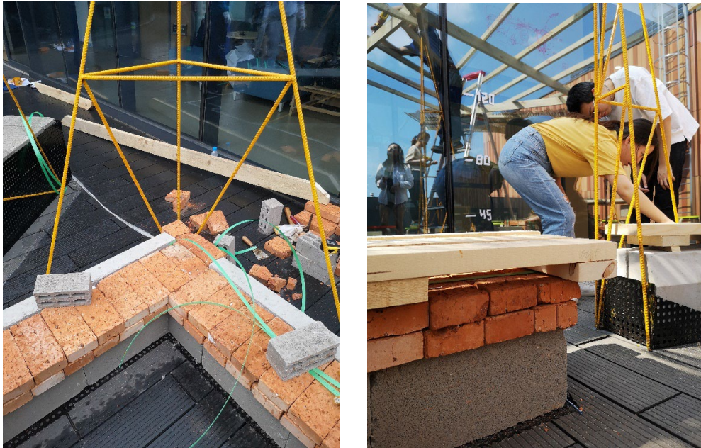
Figure 1,2. Construction process. Source: Sofia Quiroga 2018*
