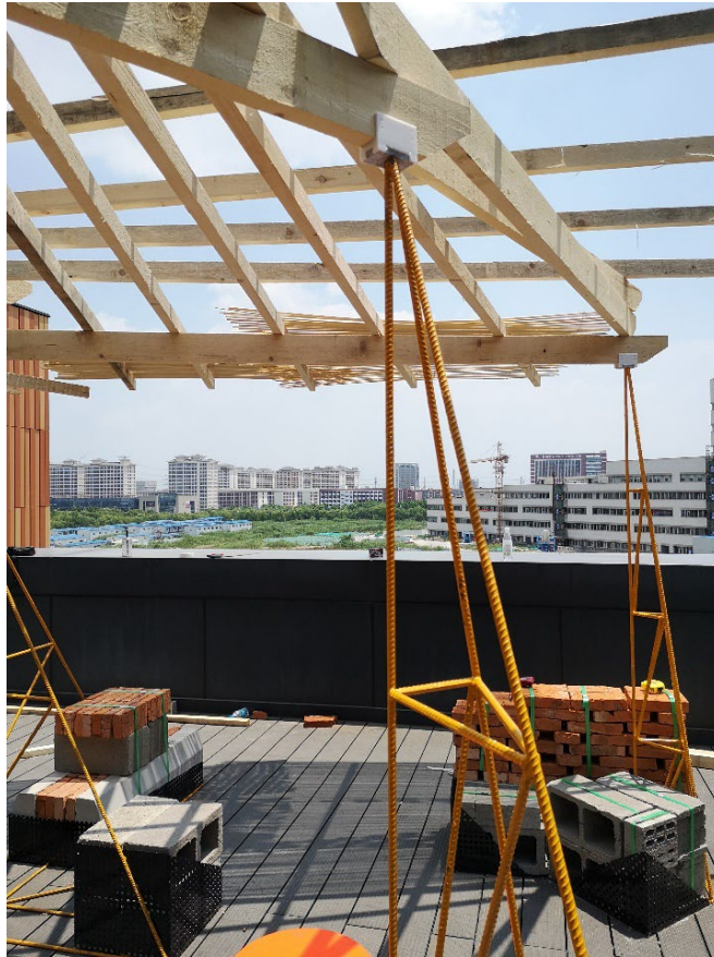
Figure 4. Construction process. Source: Sofia Quiroga 2018*
