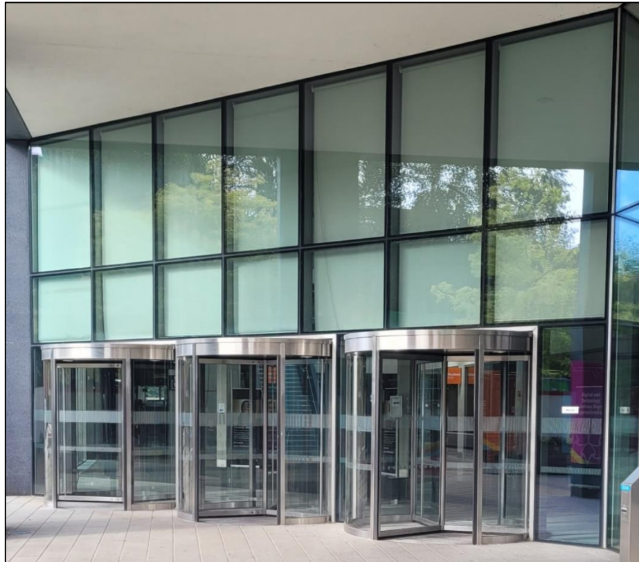
Figure 3.13 The three revolving doors for the main entrance to the Business School.
