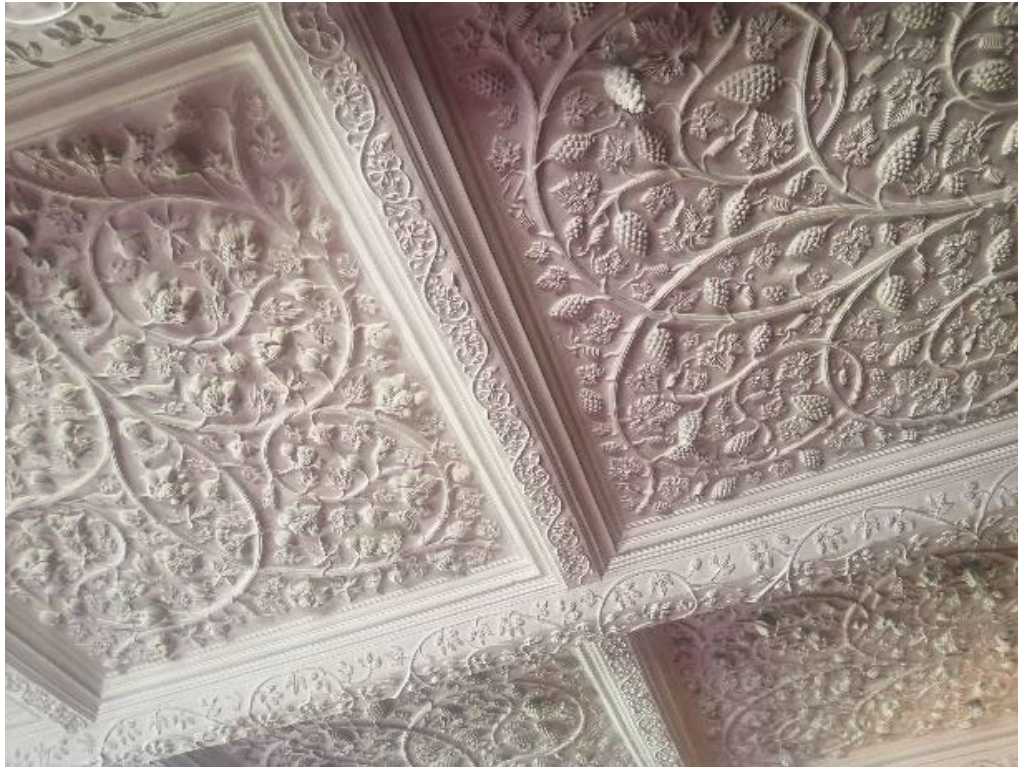
Figure 34: A section of Speke Hall's oak parlour ceiling stuccowork.
