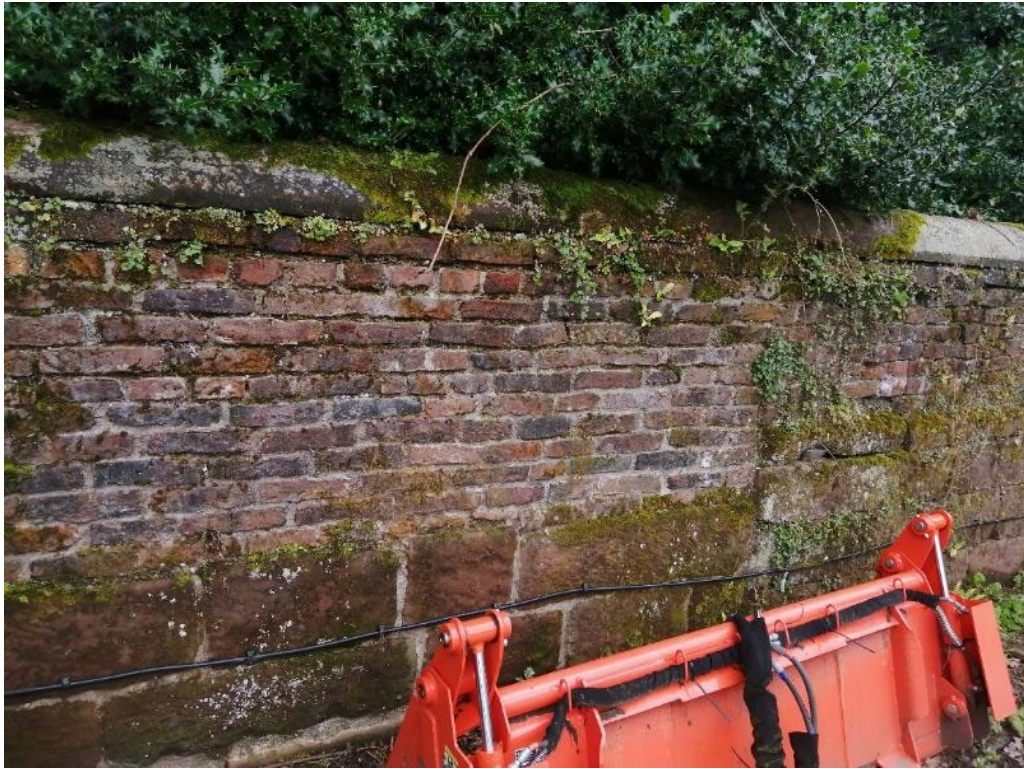
Figure 35: A section of the seventeenth-century brick wall at Speke.
