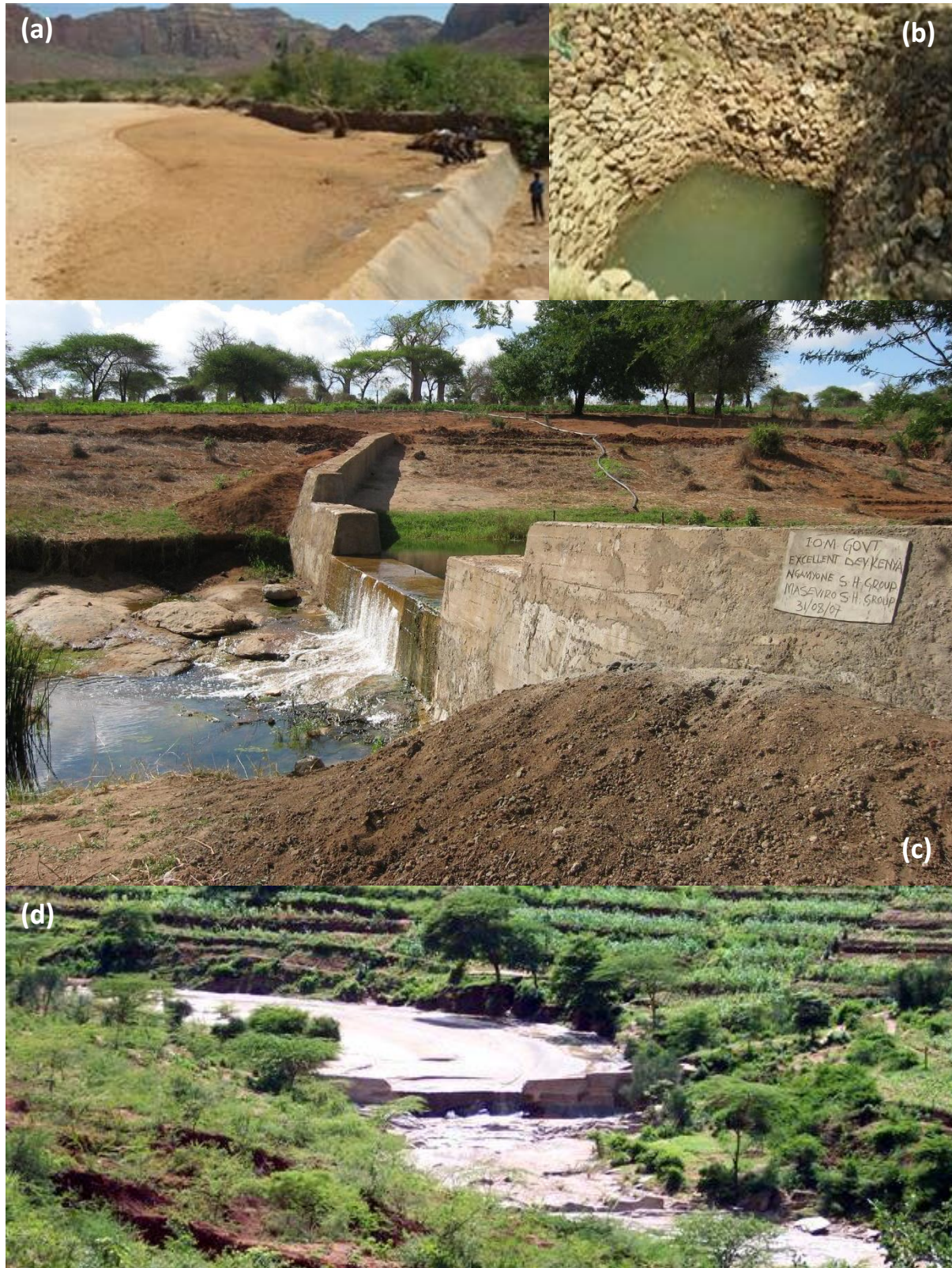
Figure 2 - Pictures of sand dams: (a) sand dam in May Gobo (Ethiopia) and scoop holes (b); (c), (d) sand dams in Kenya. Sources: (a) and (b) – photo -by Lorenzo Villani; (c) and (d) Excellent Development - (CC BY-NC-ND 2.0)
