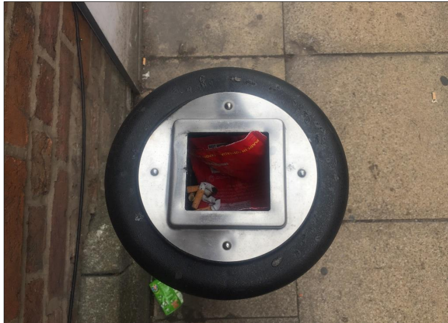
Figure 4.13: Cigarettes and Food Wrapper dropped into broken gap of Bollard [Author's own image, 2018]
