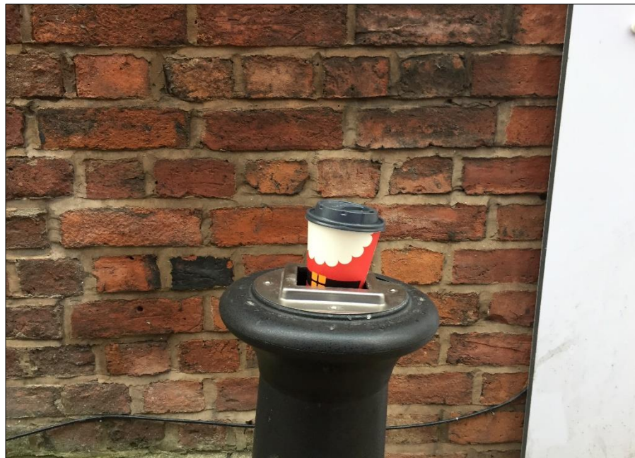
Figure 4.14: Cup dropped into broken gap of Bollard [Author's own image, 2018]
