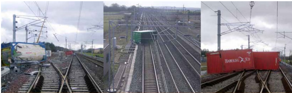
Figure 1: Detached containers blown from flatbed freight wagons travelling along the West Coast Mainline, UK, on the 1st March 2008 (RAIB, 2009).
