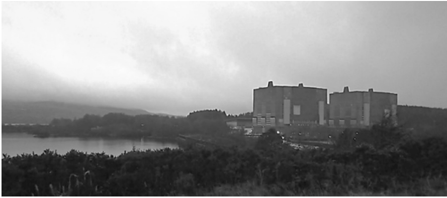
Fig. 5. View of Trawsfynydd 'cathedral like' reactor buildings from viewing platform next to site (Source: researcher's own, December 2017).
