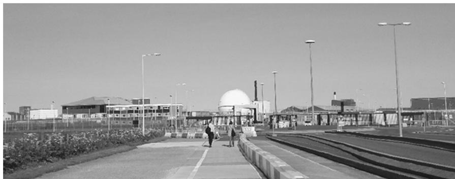
Fig. 4. View of entrance to Dounreay site with the iconic 'Sphere' housing the decommissioned reactor, (Source: researcher's own, July 2017).
