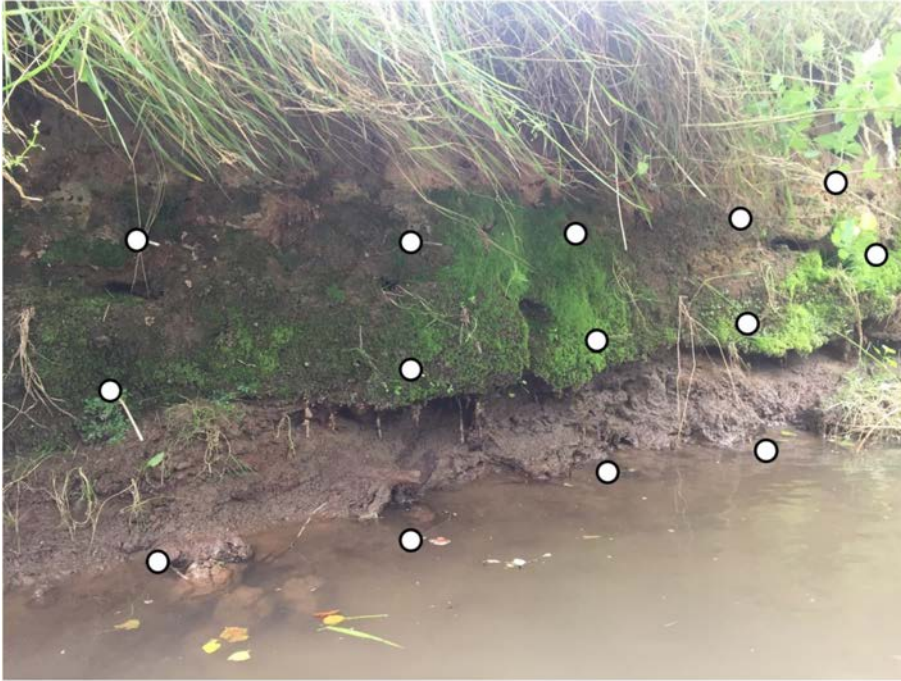
FIGURE 5 An undercut bank on the River Bain. The spacing of the erosion pins (denoted by circles) was often too coarse to detect these local processes which lead to large-scale collapses. (NB: Photograph taken during low flow conditions for clarity of bank morphology) [Colour figure can be viewed at wileyonlinelibrary.com ]
