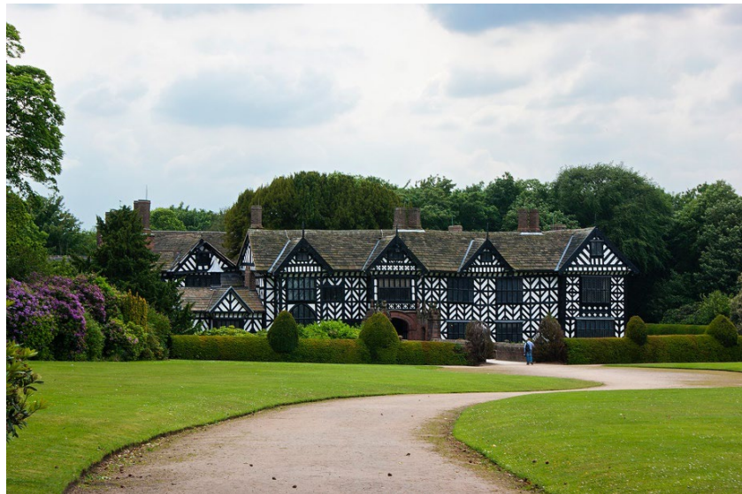
Fig. 2. Speke Hall, Lancashire, home of the Norris family. Exterior of north range. Image courtesy of Ian Greig.
