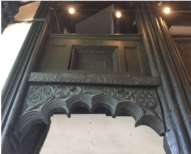
Fig. 11. Door arches, with hexafoil carved motifs, in the 19 th century hall woodwork at Salmesbury. These are the 16 th century arches that were over the entrances to buttery, kitchen and pantry. Image author's own.
