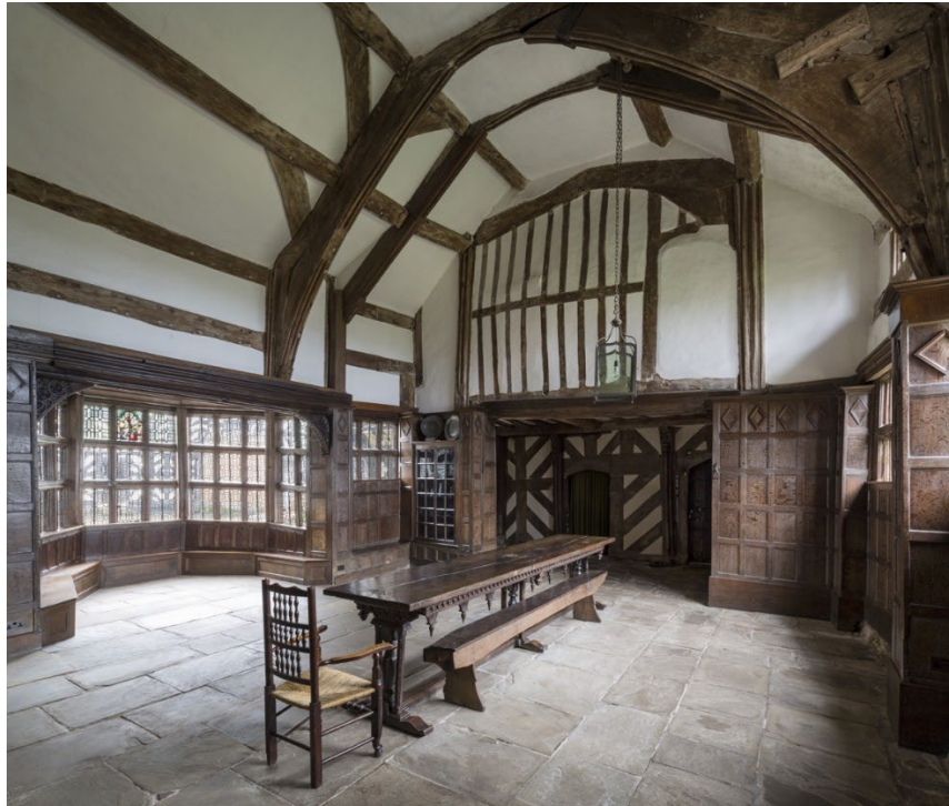
Fig. 8. Great hall with filled in doorway linking the bedchambers at the east end of the hall to those on at the west end, which were accessed via another door still visible today. Image courtesy of National Trust Images
