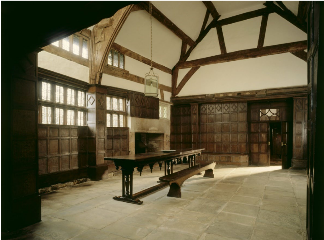
Fig. 7. Great hall showing the cut off joists for the inserted first floor and the entry to the parlours. Image courtesy of National Trust Images.
