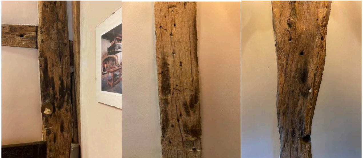
Fig. 6. Burn marks in the kitchen at Martholme, another of the Hesketh properties. Photos author's
