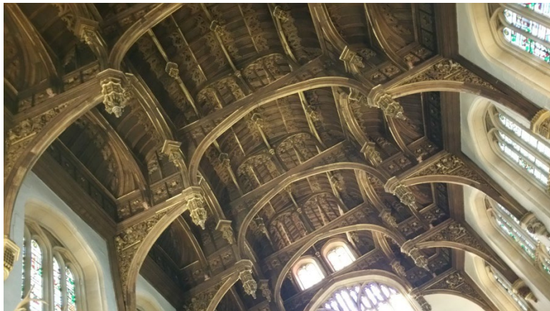
Fig. 7. All'antica hammerbeam ceiling at Hampton Court. Image courtesy of J. Rennocks [CC-BY 4.0]
