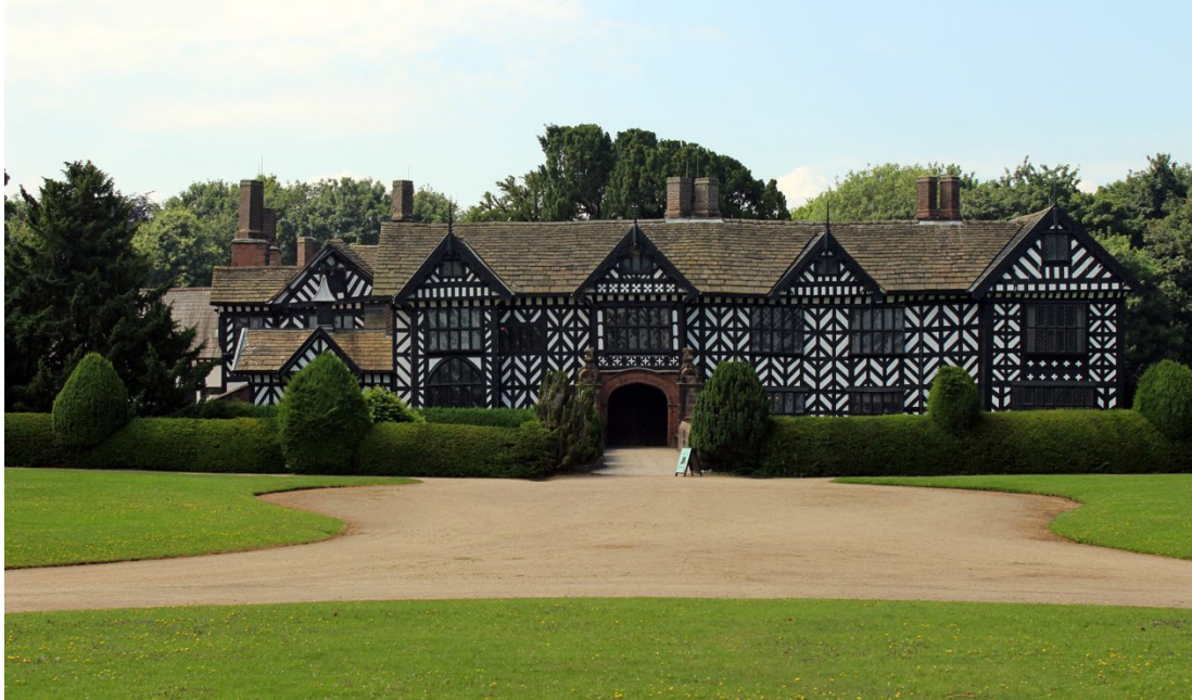
Fig. 1. The north wing at Speke showing the gateway through to the enclosed courtyard, from which guests would enter the Great Hall. To the left of the photograph is some of the service wing to the east housing the kitchens, dairy, the remains of the old chapel (hinted at by the arched window) and the various outbuildings of Speke's service courtyard. Image courtesy of National Trust Images.
