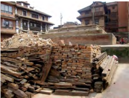
Bricks and Timber salvaged from the temple stacked at the site
