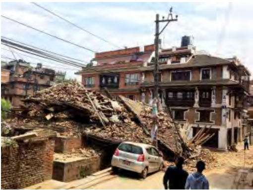
The remains of the Radha-Krishna Temple at Swotha, after the earthquake of 25 April 2015 [Credits: Kathmandu Valley Preservation Trust]
