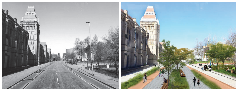
Figure 14 Before and after street views according to our future visions (Source: Author)
