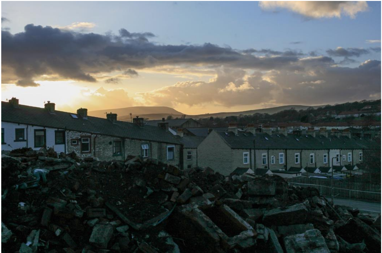
Fig. 17 Demolition Street , rubble with Pendle Hill in the distance (See Appendix E: Tittley 2009).
