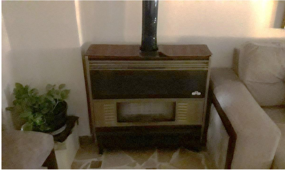
Figure 47. Electric heater in the girl's bedroom
