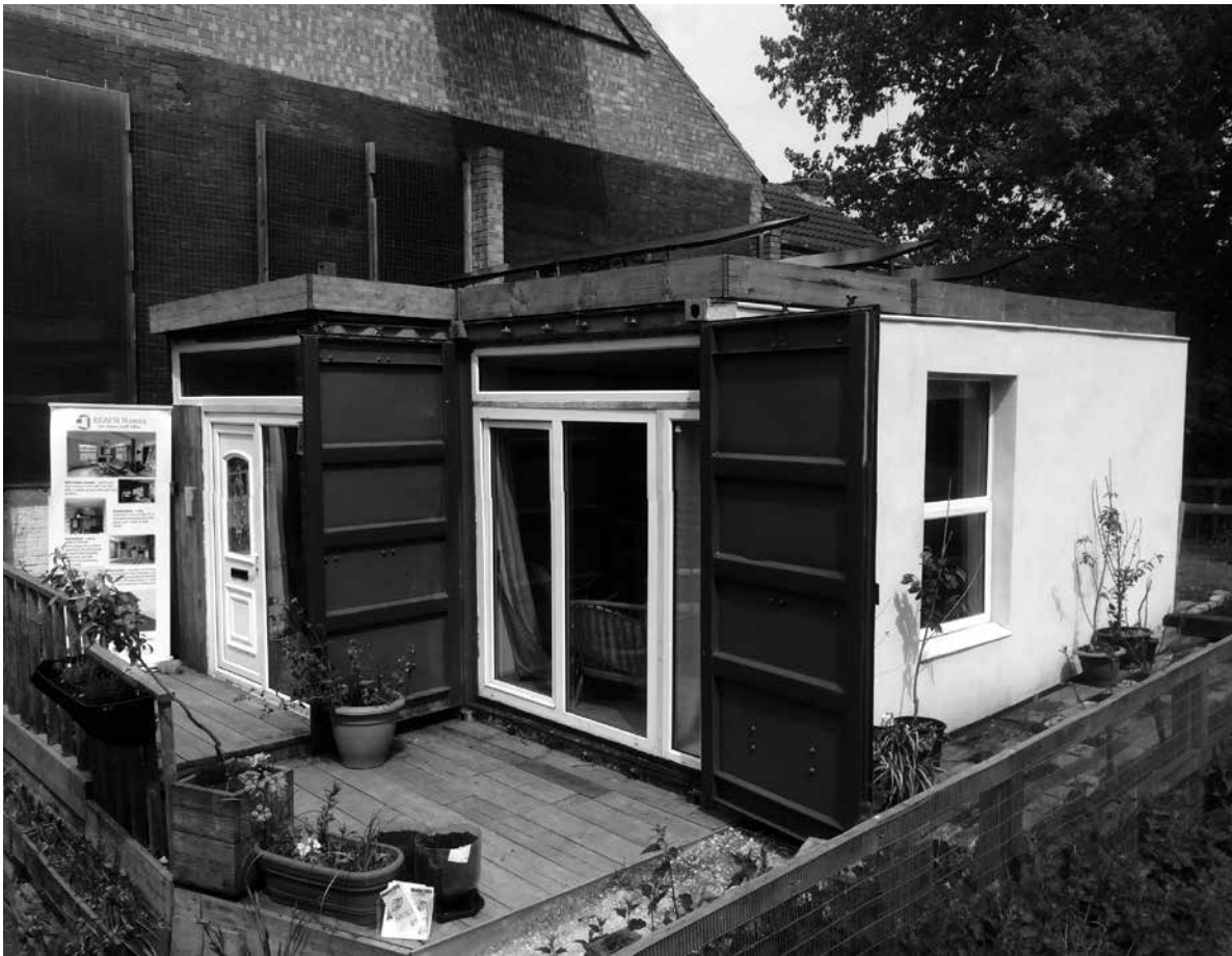
1 Exterior of REACH Homes prototype.
