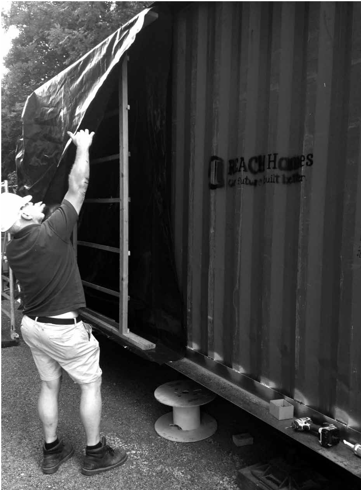
3 Applying DPM and secondary structure to the shipping container.
