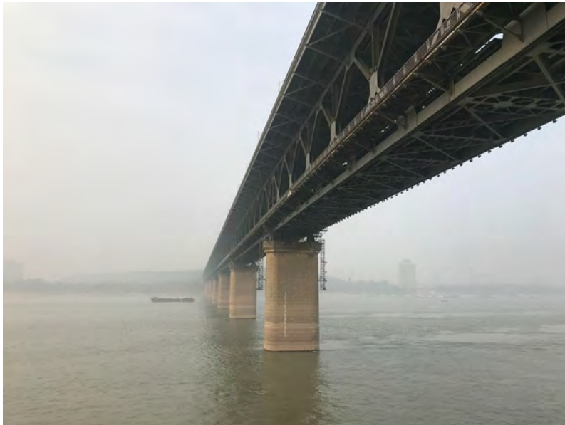
Fig. 26. Sailor, L., Wuhan Yangtze River Bridge, 2019 [Photograph]
