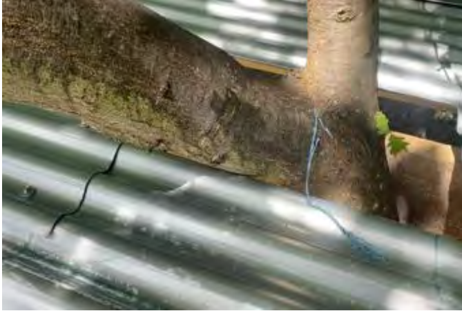
Figure 41: Tree Scaping on Roof (Source: Steve Pool 2020)
