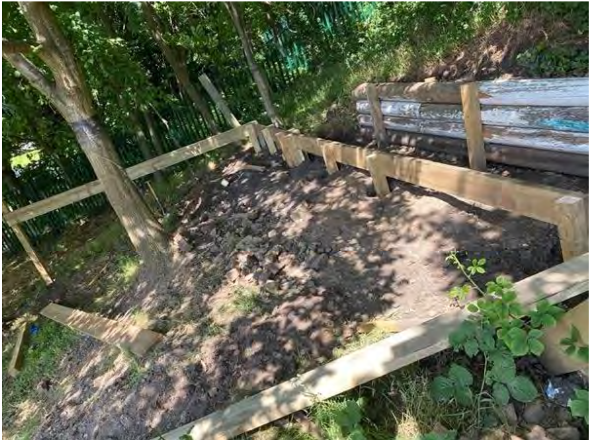
Figure 47: Building Platform 2 (Source: Steve Pool 06:2020)
