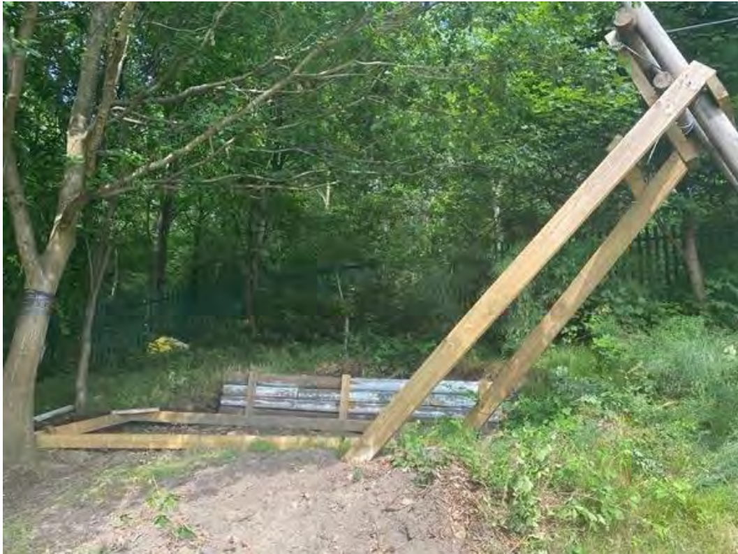
Figure 45: Building Platform 1 (Source Steve Pool 03:2020)
