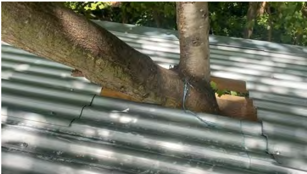
Figure 53: Building the Platform 8 (Source: Steve Pool, 09:2020)
