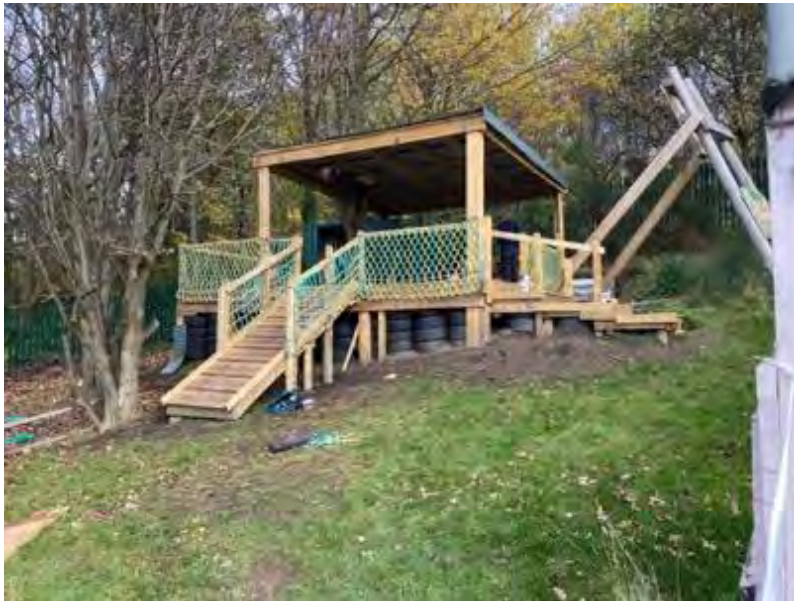
Figure 3: Platform nearing completion (Source: Steve Pool 11:2020)
