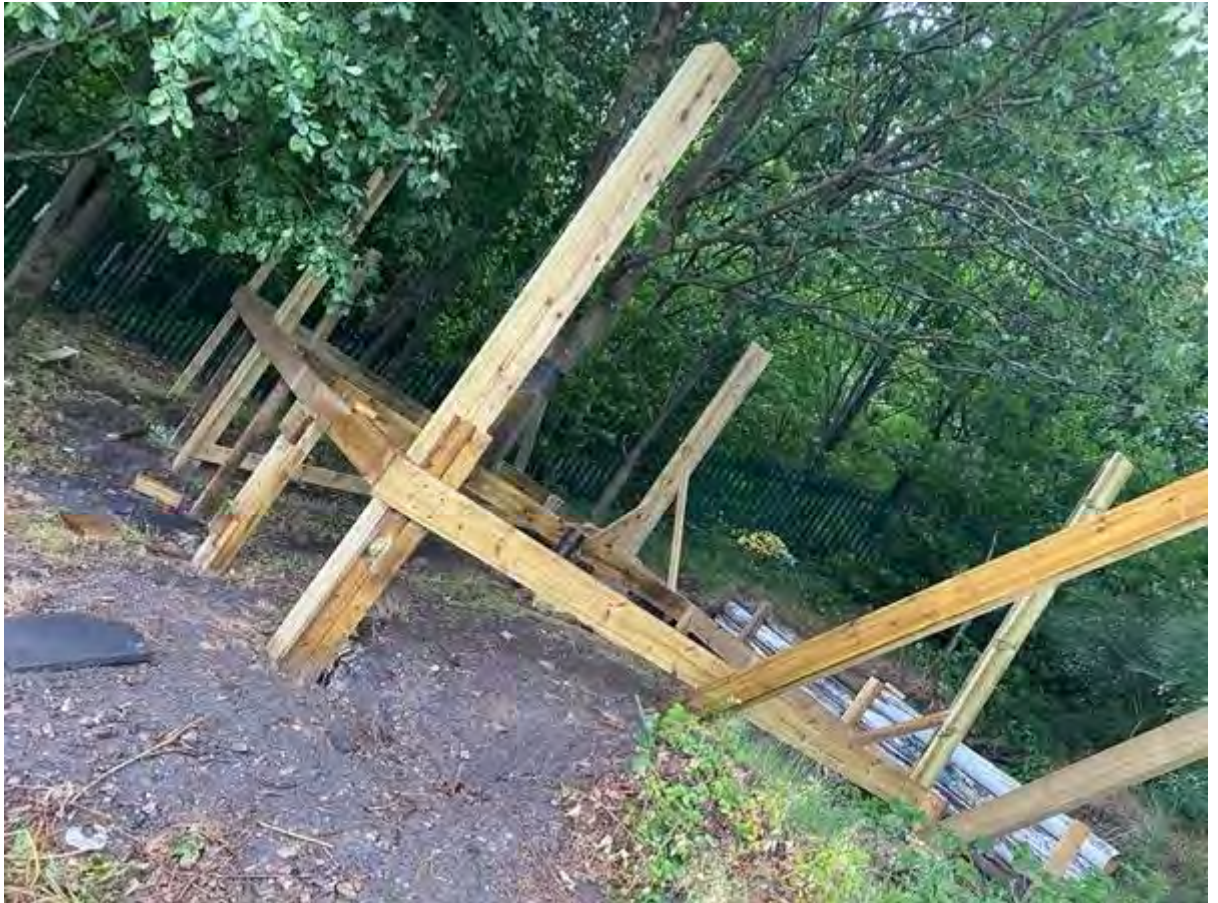
Figure 48: Building Platform 3 (Source: Steve Pool 05:2020)
