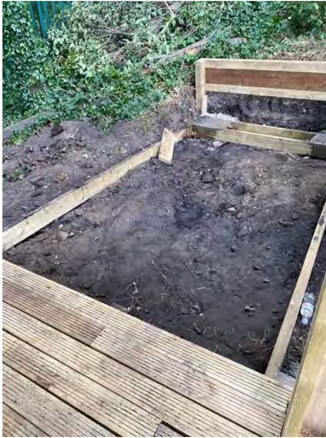
Figure 54: Building the Platform 9 (Source: Steve Pool, 09:2020)
