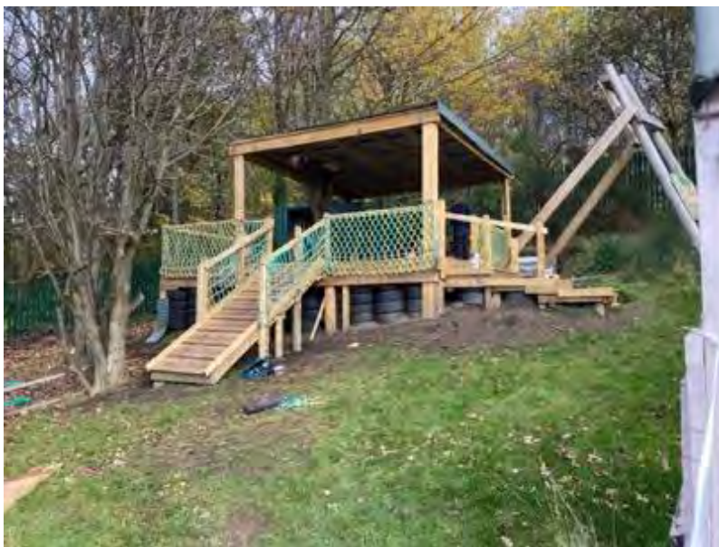
Figure 36: Platform nearing completion (Source: Steve Pool 11:2020)
