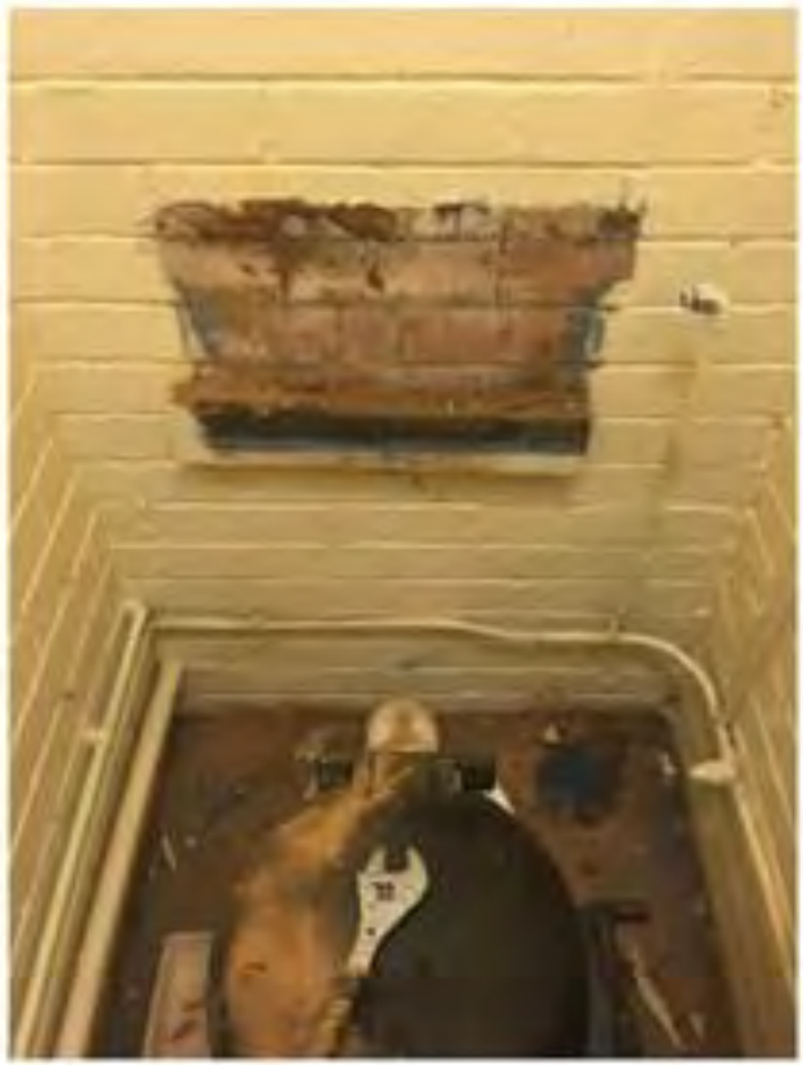
Figure 33: Removing the Old Flush Tank (Source: Steve Pool 01:2019)
