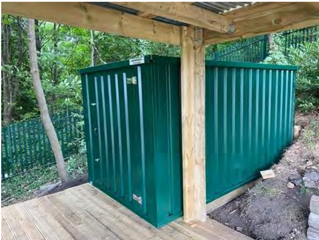
Figure 55: Building the Platform 10 (Source: Steve Pool, 10:2020)
