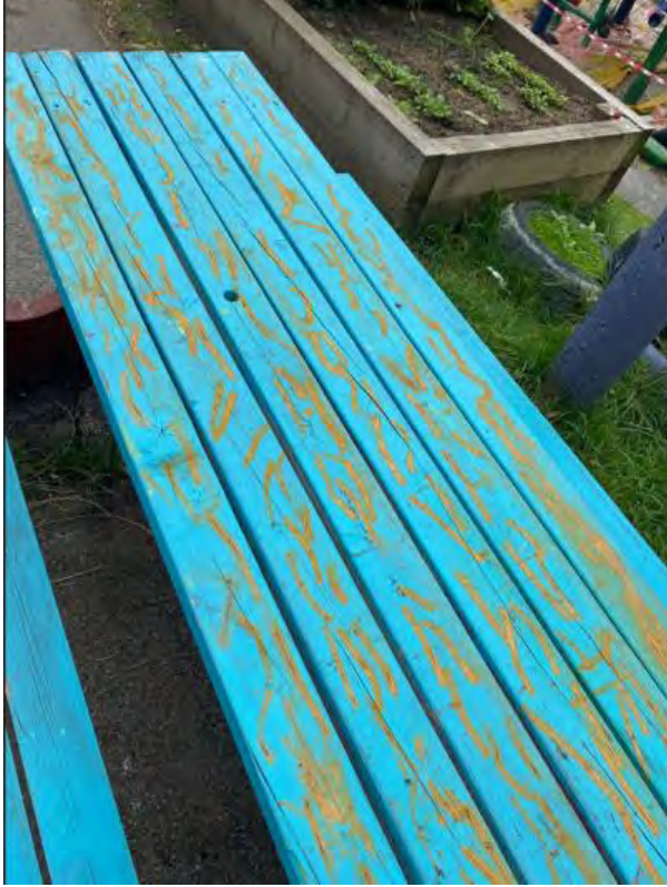
Figure 42: Marks Left by Rusting Nails (Source: Steve Pool 08:2020)
