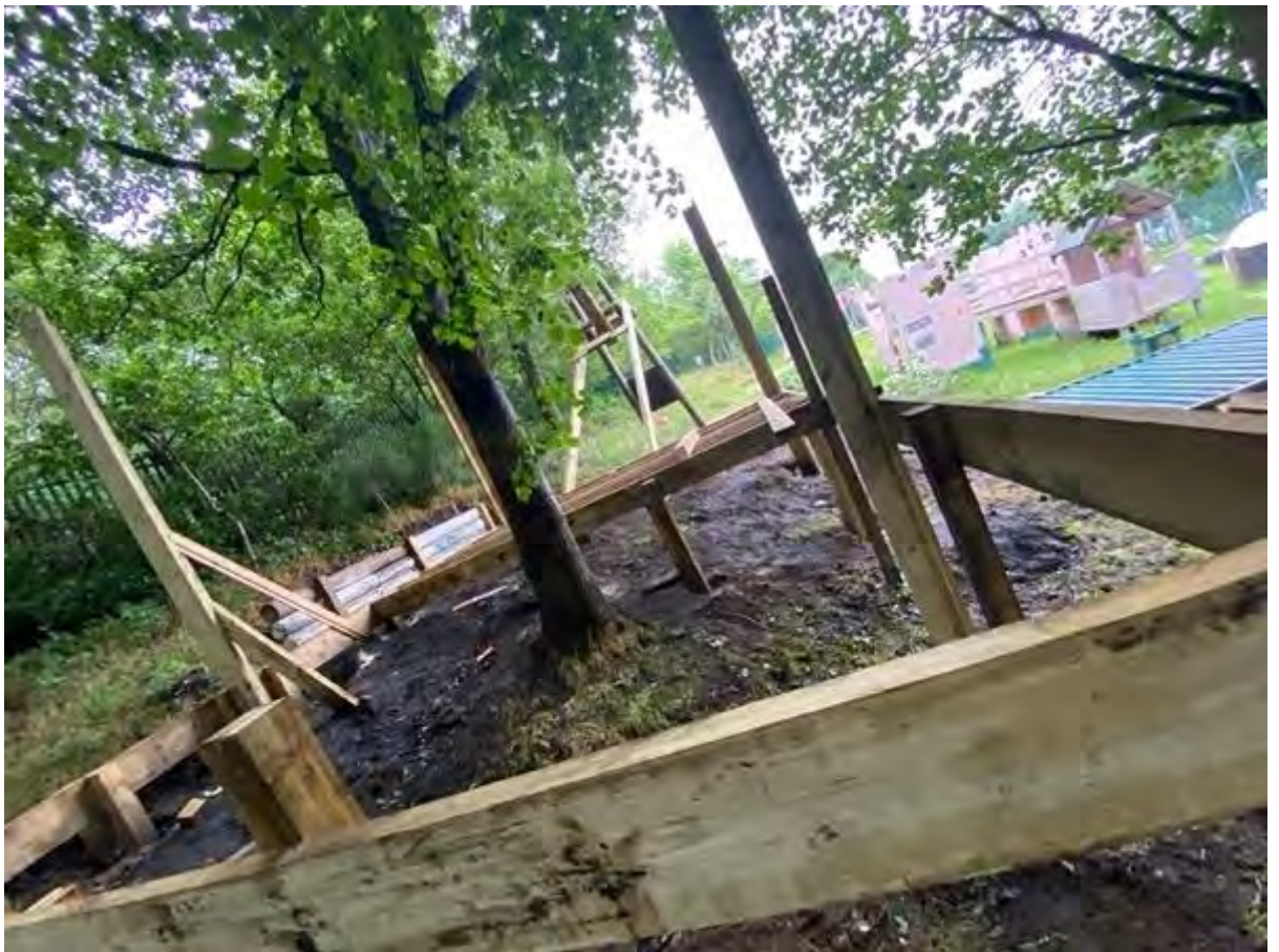
Figure 49: Building Platform 4 (Source Steve Pool 05:2020)
