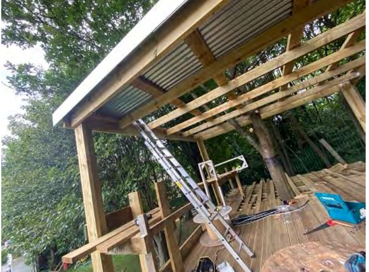
Figure 52: Building the Platform 7 (Source: Steve Pool, 07:2020)
