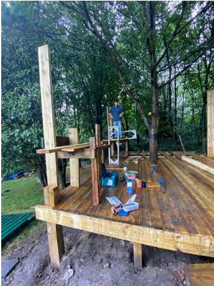
Figure 51: Building the Platform 6 (Source: Steve Pool 07:2020)
