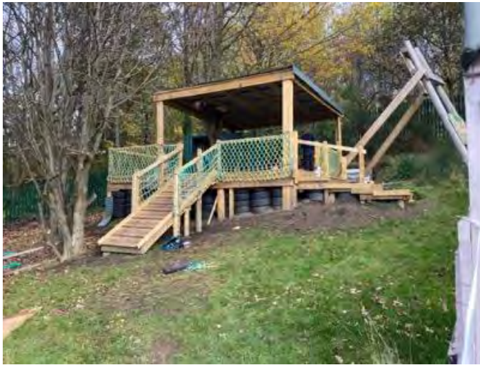
Figure 59: Platform Nearing Completion (Source: Steve Pool 09:2020)
