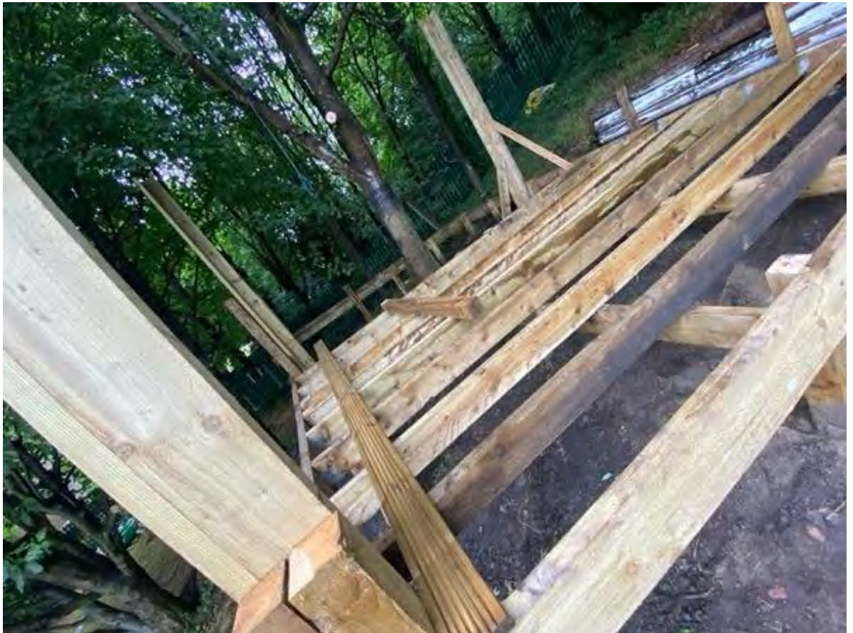
Figure 50: Building the Platform 5 (Source: Steve Pool, 06:2020)
