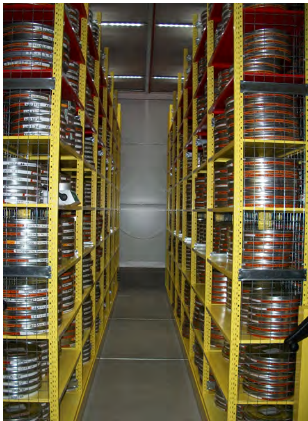
Fig.90. The newly built vaults at the BFI, Gaydon. In the event of combustion of nitrate film the sides of the vaults blow out into the trench. The reinforced concrete ensures only one vault of film reels would be lost due to fire in a single vault.
