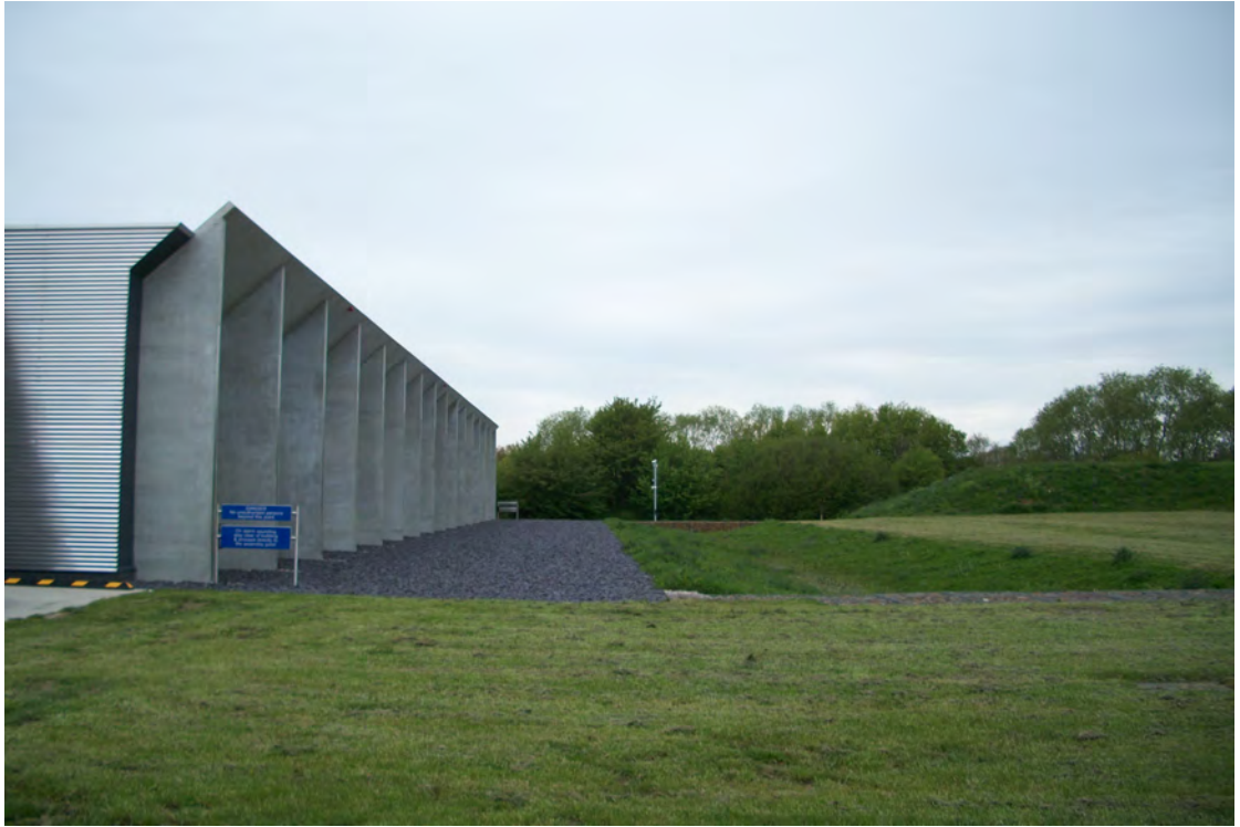
Fig.90. The newly built vaults at the BFI, Gaydon. In the event of combustion of nitrate film the sides of the vaults blow out into the trench. The reinforced concrete ensures only one vault of film reels would be lost due to fire in a single vault.
