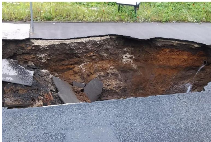
Figure 7: Sinkhole picture 1 [Source: (News, 2015)]
