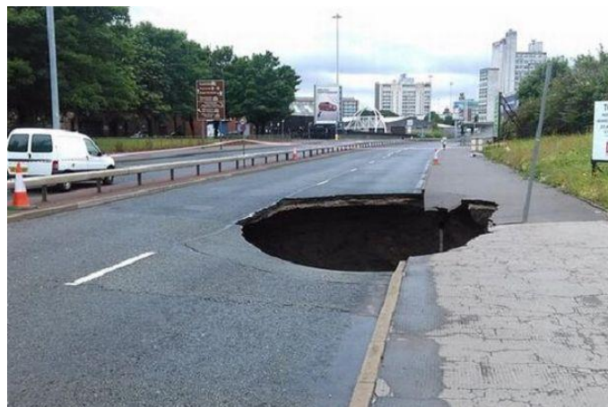
Figure 8: sinkhole picture 2 [Source: (News, 2015)]
