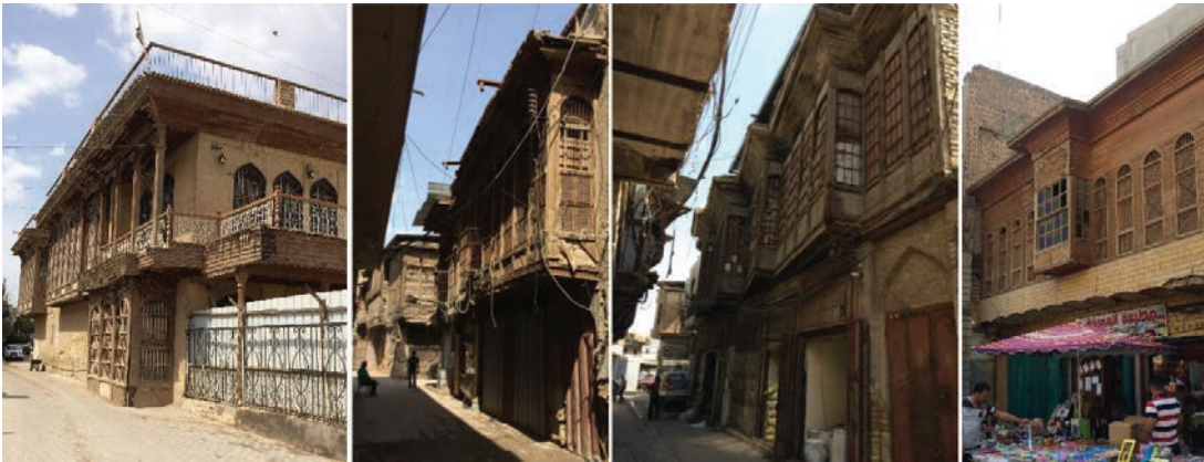
Fig. 12 - Shanasheel Filters Light, Increasing Ventilation, and Allows Looking Outside without Being Seen. Source: Author 2020.
