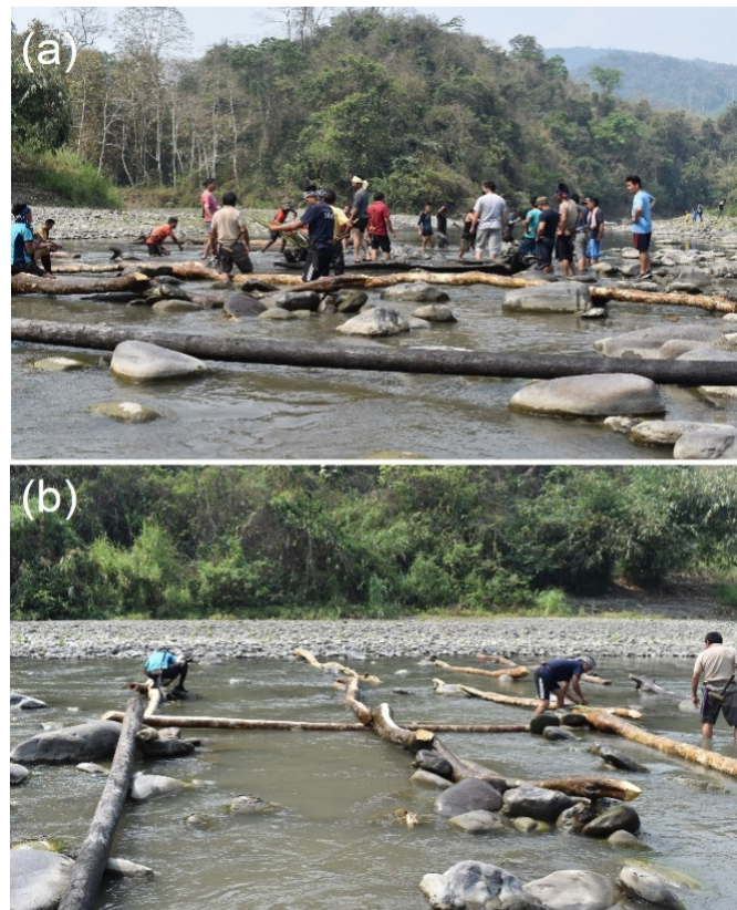
Figure 5. (a,b) Construction of wood platforms across the river for the pounding of M. pachycarpa for community fishing in Nagaland, Northeast India.
