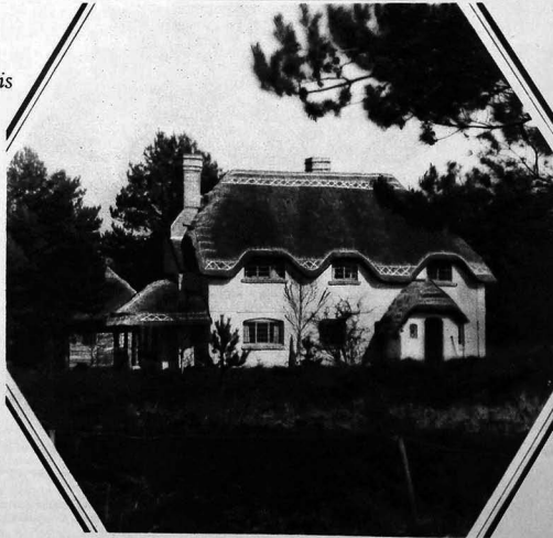
FIG. 2 "Other People's Homes," first page of Photogravure Supplement showing Cottage designed by R. F. Wells and built by Tiles & Potteries Ltd., published in Modern Home (September 1929): 29.
