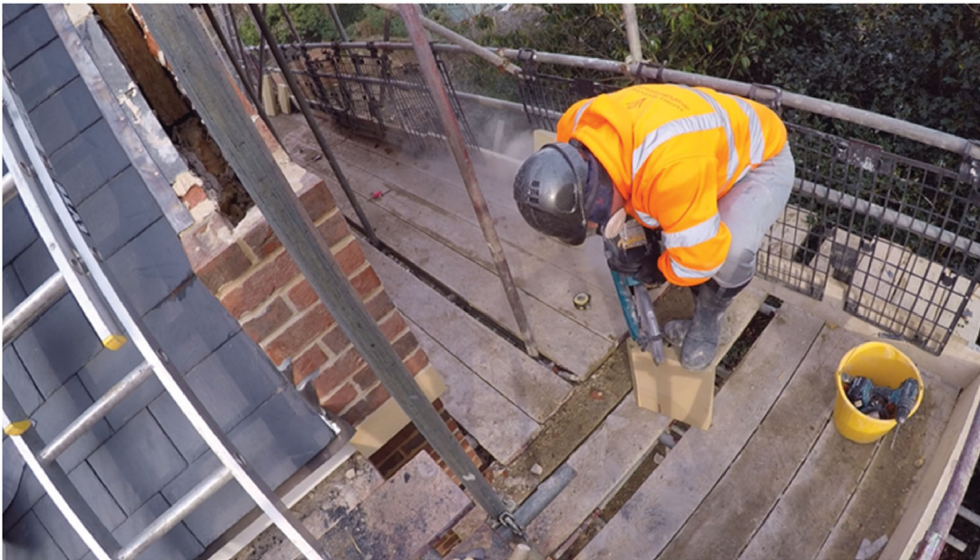
Figure 1. The bricklayer cuts the coping stone with the petrol disc cutter. This is a still from video footage taken by the principal author using a handheld camera.
