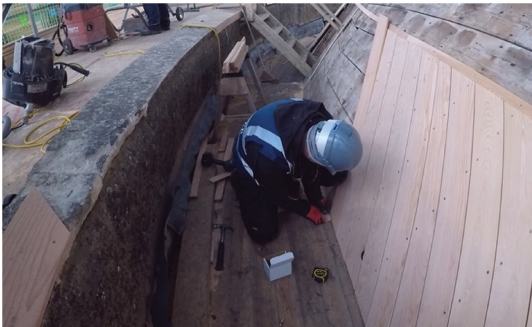
Figure 2. The carpenters scribe the cladding before cutting the bevel.
