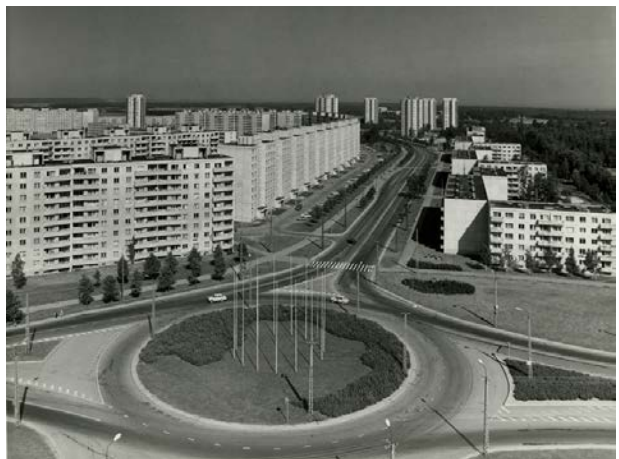
Figure 11: Construction of new residential buildings in Mustamäe, Tallinn (Source: Kuznetsov: online)
