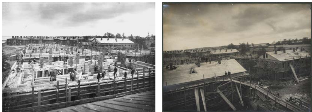
Figure 305–306: The construction of residential buildings in progress on central lines (Source: The collection of the Estonian Maritime Museum: online)
