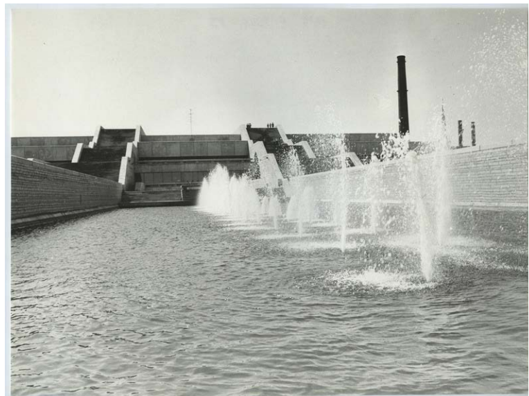
Figure 49: The north side of Linnahall with water cooling pools (Source: ETA, 1980–1990: online)
