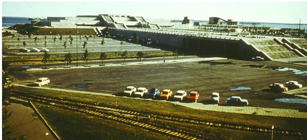
Figure 30: The building initially functioned as a railway bridge for pedestrians (Source: Linnahall: online)
