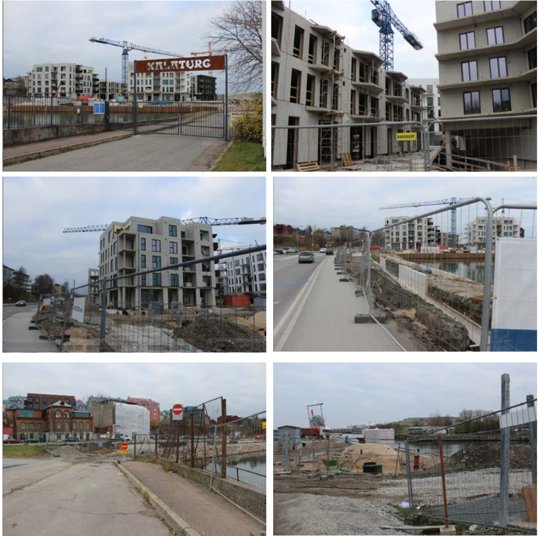
Figures 665–670: The mixed-use development in progress (Source: Kurik, 2020)
