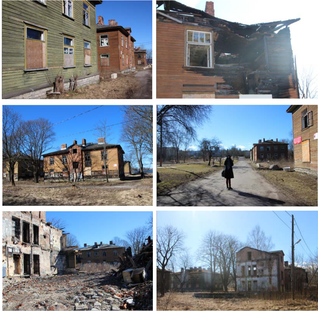
Figures 396–401: The lower lines continue to be a mix of buildings that are relatively intact and buildings that will most likely be lost. The brick staircases visible on lower images will be preserved and later used as the core of new buildings that will replicate the historic structures (Source: Kurik, 2017)
