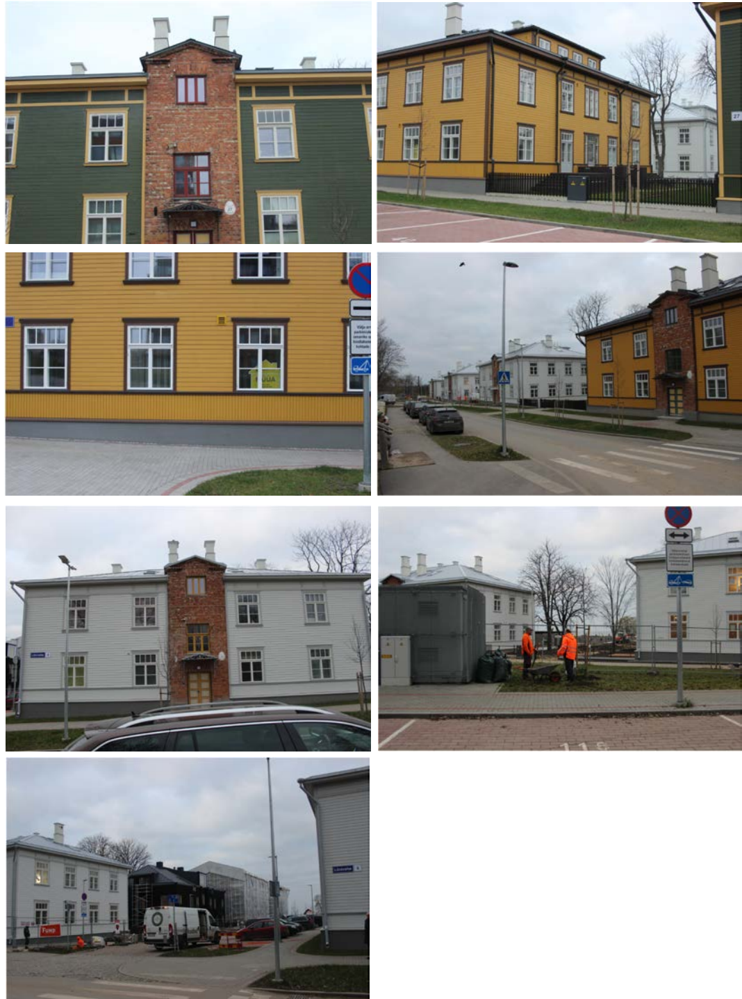
Figures 464–470: New buildings have emerged around preserved central staircases. While historically these buildings housed very small apartments for workers, the new ones, while looking very similar externally, have been redesigned to accommodate contemporary needs (Source: Kurik, 2020)
