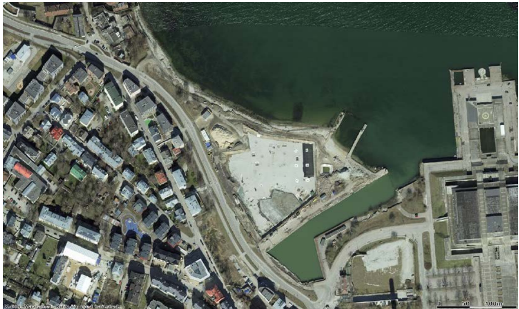
Figure 501: The site in 2019 – the construction of the new mixed-use area has started (Source: Republic of Estonia Land Board: online)
