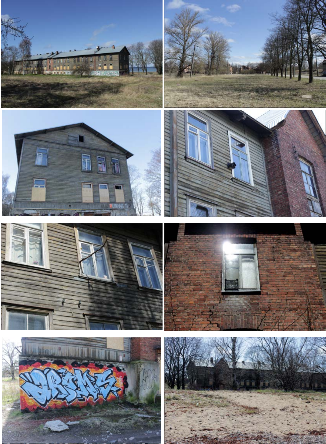
Figures 366–373: The burnt buildings visible in the site visit photography from 2013 have been cleared and this area appears somehow the clearest and best preserved despite the boarded-up windows. It looks like this building could be restored in its original form (Source: Kurik, 2016)
