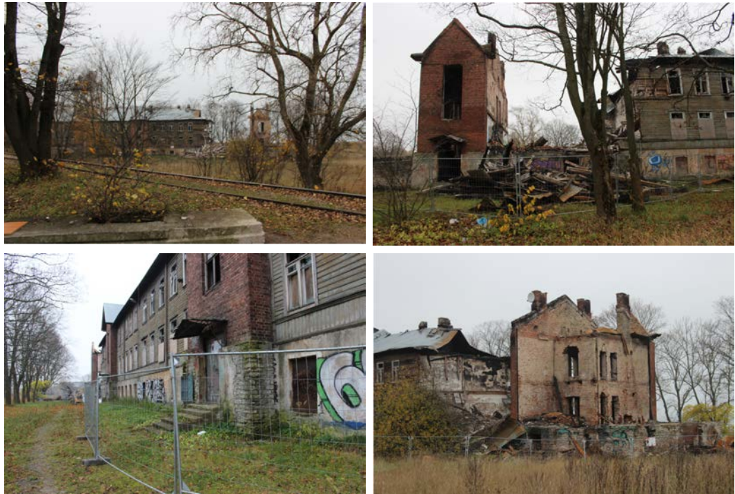
Figures 428–431: There has been another fire and the long building that has stood relatively intact on the central lines has been significantly damaged (Source: Kurik, 2019)
