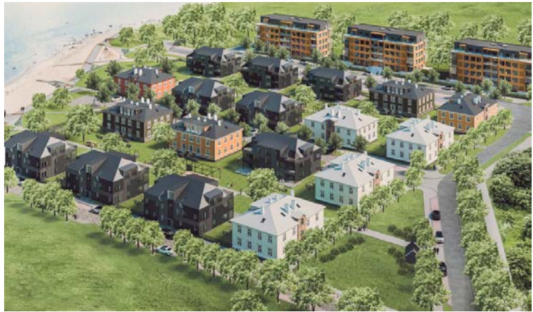
Figure 324: A vision for the second typology in the former specialised workers' housing area (Source: Fund Ehitus/Apex Architects: online)
