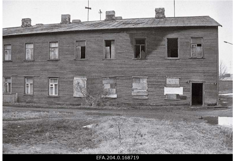
Figure 294: A residential building in Kopli in February 1989 (Source: Truuväärt, 1989: online)
