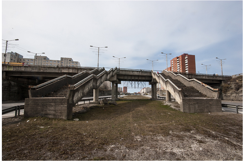
Figure 17: Steps leading to a never realised tramline in Lasnamäe, Tallinn (Source:Maran, 2014: online)
