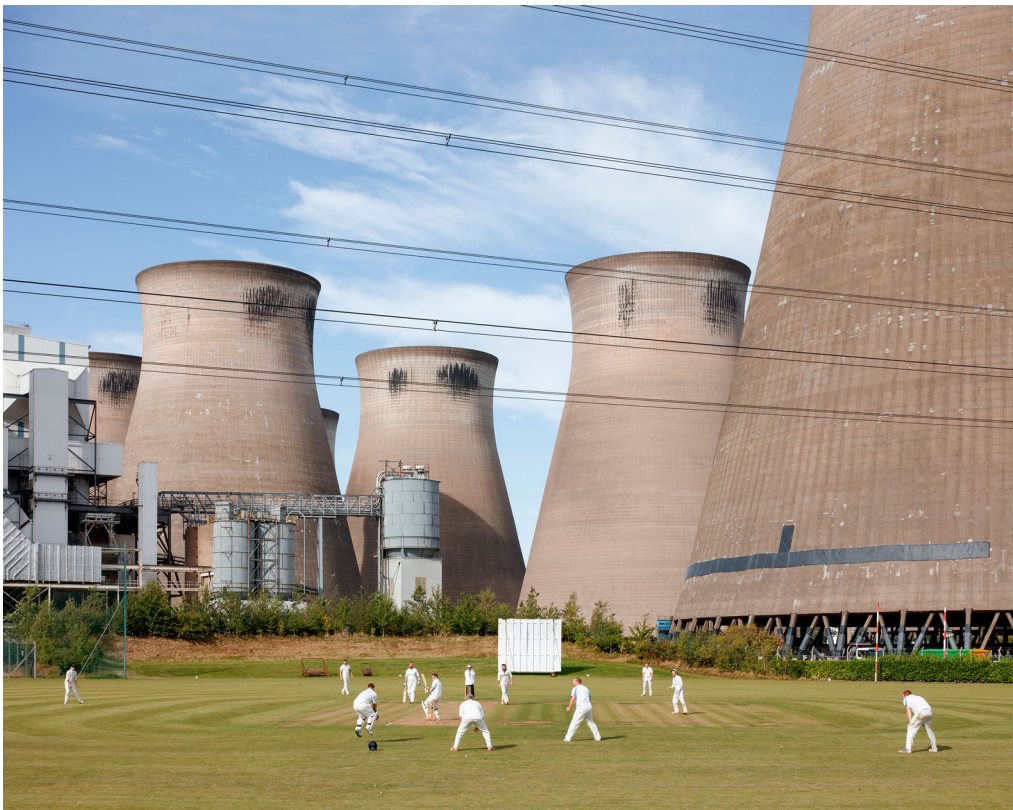
Figure 1. The last cricket match at Ferrybridge C Power Station in West Yorkshire before the demolition of the cooling towers in 2019 © Luke O’Donovan.
