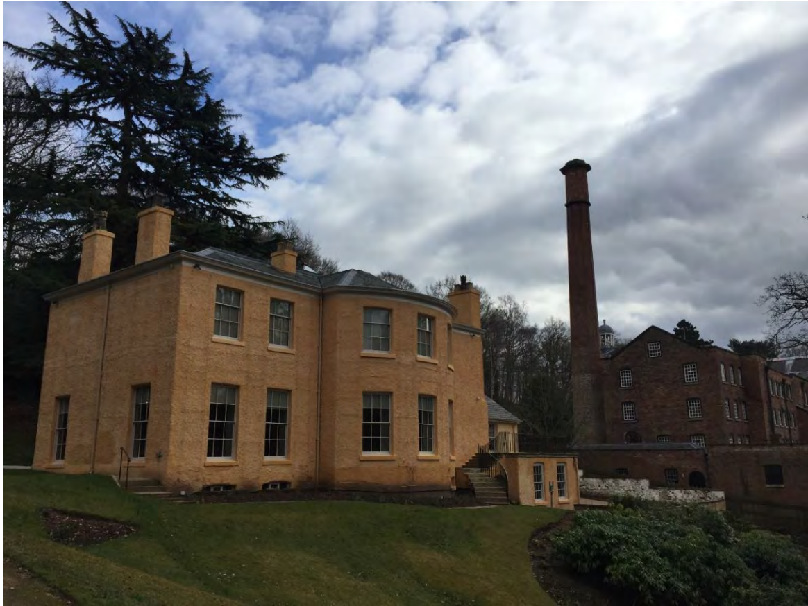
Figure 2.9: A rear view of Quarry Bank House and the mill. The service wing, which was demolished in the 1960s, was on the right of the house and it ran all the way up to the boundary wall with the mill. (T. McGrath, 2018)
