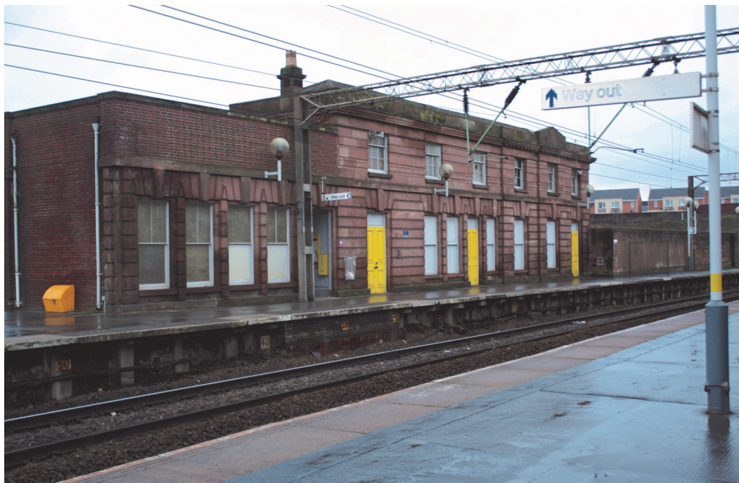
Figure 12: Edge Hill station (1836), south side buildings.
