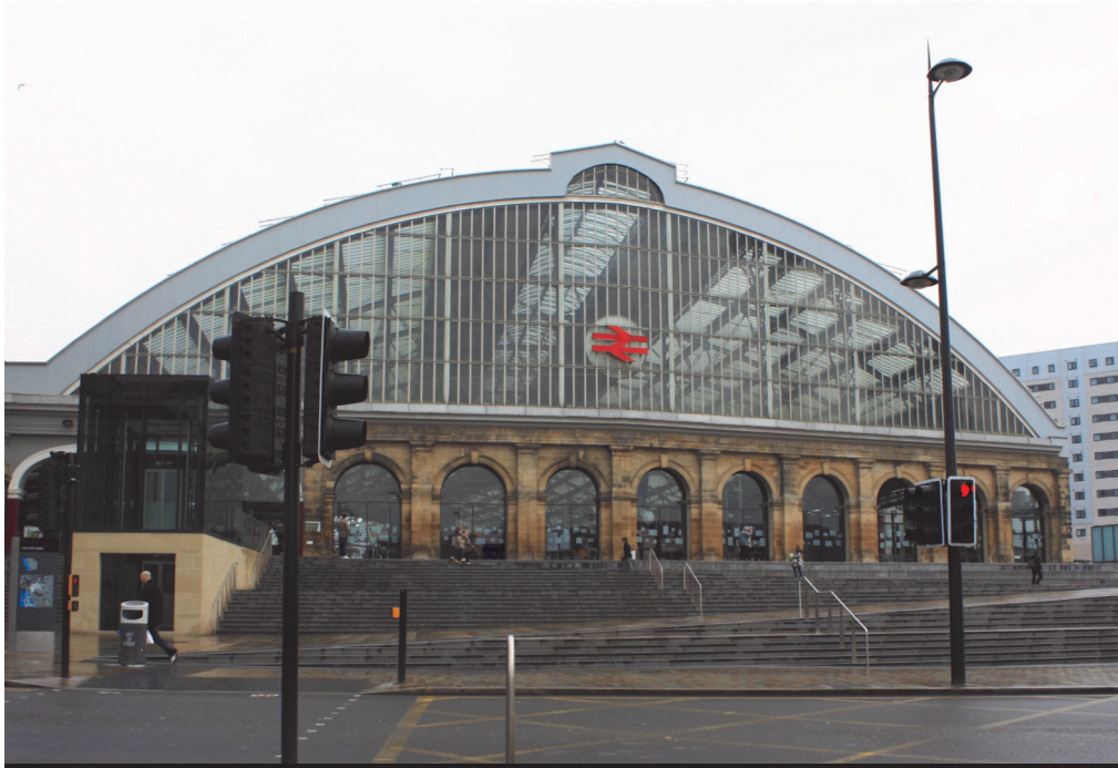
Figure 13: Entrance to Lime Street Station.
