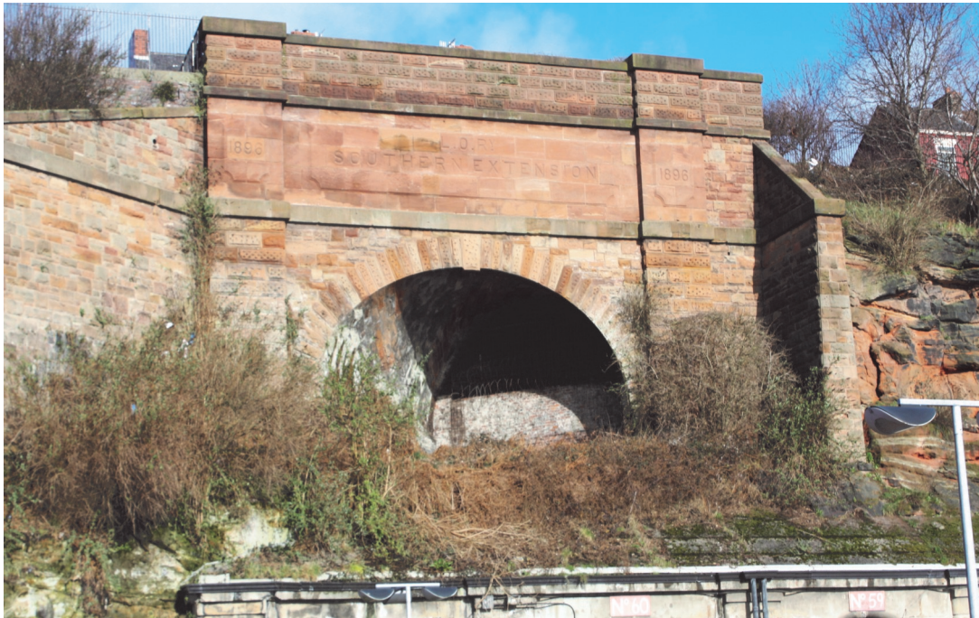
Figure 15: Portal to the Dingle tunnel section of the former Overhead Railway.
