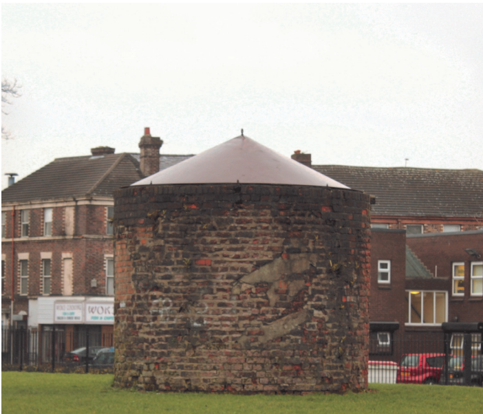
Figure 9: Ventiation shaft for the Victoria tunnel, Helena Street.
