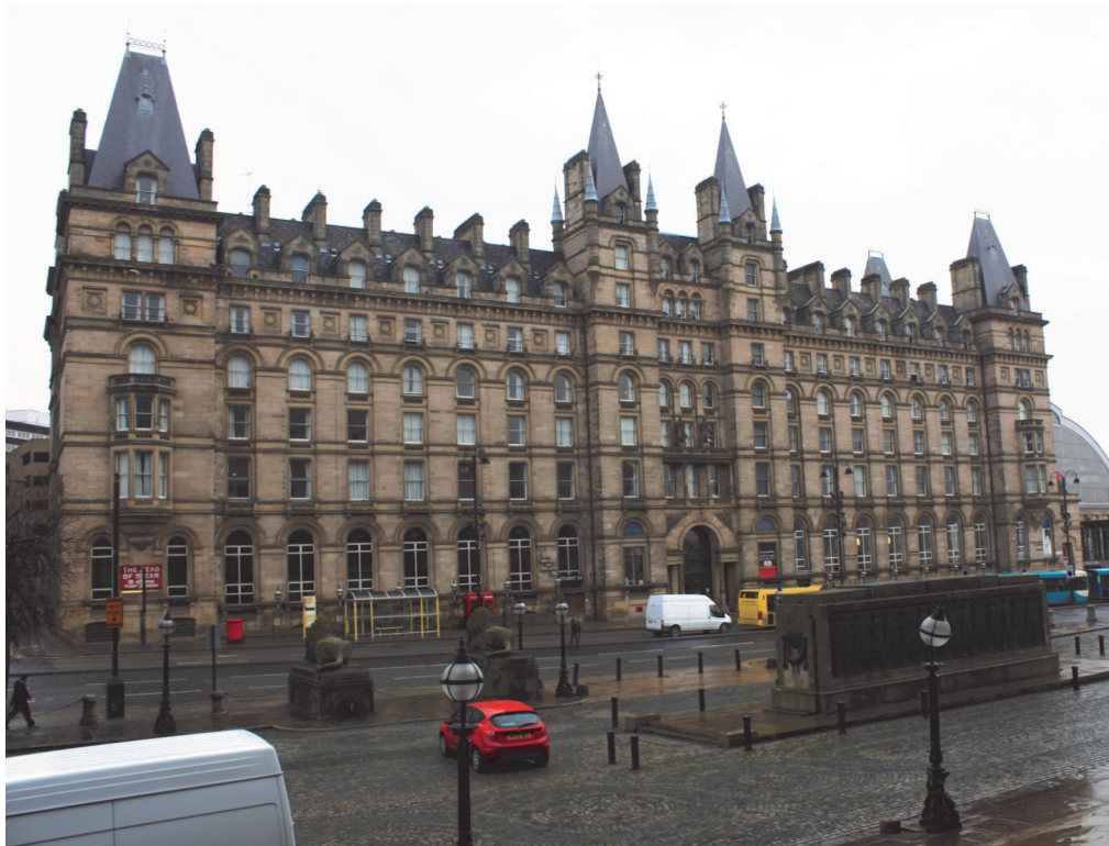
Figure 14: Lime Street Chambers (1867) by Alfred Waterhouse
