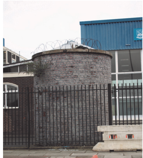
Figure 8: Ventilation shaft for the Victoria tunnel, Archbishop Blanch High School, Minshull Street.
