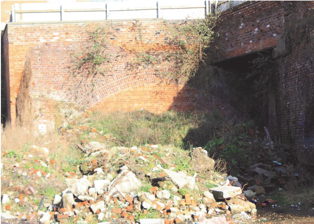
Figure 6: The western portal of the Wapping tunnel, King's Dock Street.
