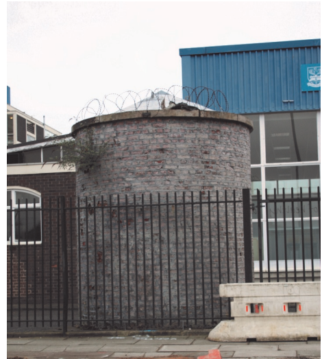
Figure 8: Ventilation shaft for the Victoria tunnel, Archbishop Blanch High School, Minshull Street.
