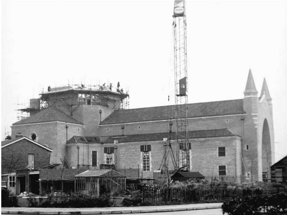
1.6 Saint Anthony's Roman Catholic Church (1960) under construction, Woodhouse Park, Wythenshawe.
