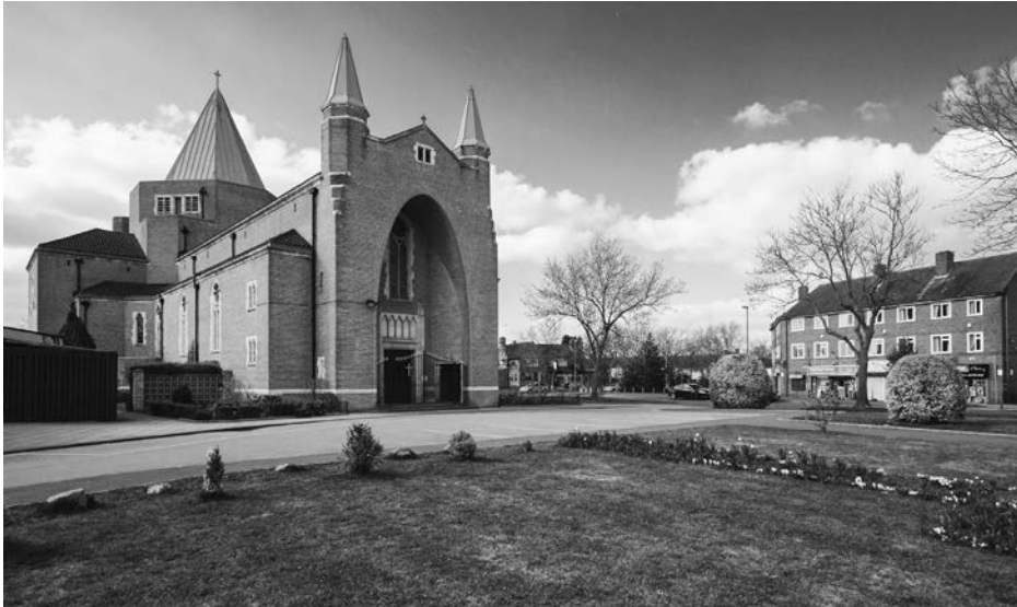
1.7. Front view of Saint Anthony's Roman Catholic Church (1960), current situation, Woodhouse Park, Wythenshawe.
