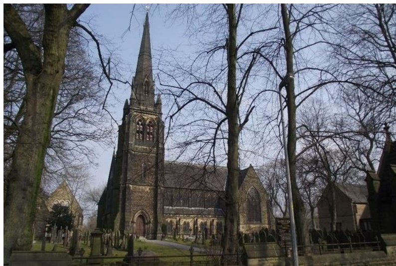
Figure 33 - Monton Unitarian Church, Salford, UK (Grade II* listed)
