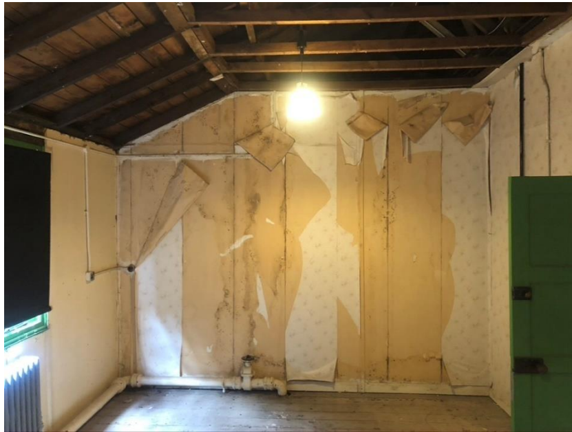
Figure 72 - Time capsule room (hut 3) remains in its pre-conservation condition
