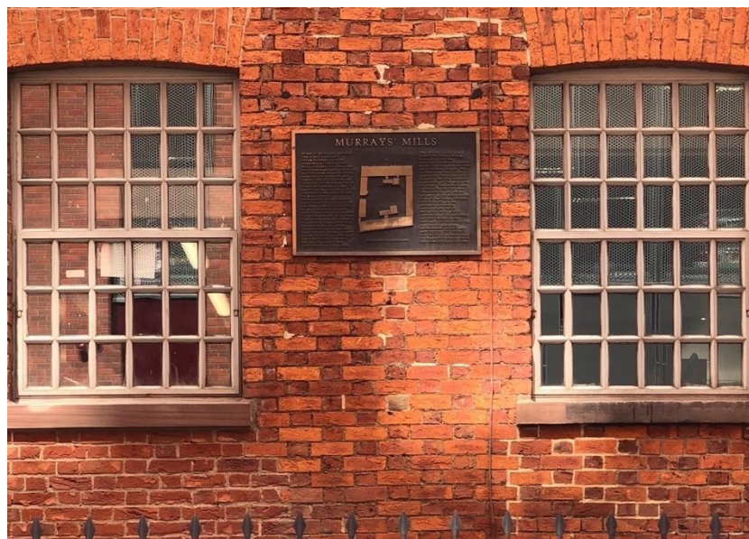
Figure 106 - Interpretation panel of the original Murrays' Mills complex, Manchester
