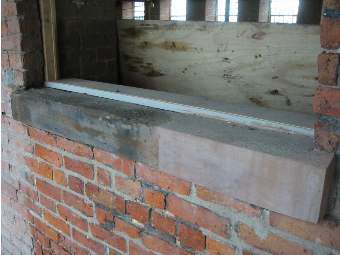
Figure 02. Isolated sandstone repair at Murrays Mills, Manchester. A restoration approach?
