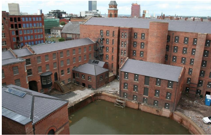
Figure 101 - Murrays' Mills, Ancoats, Manchester
