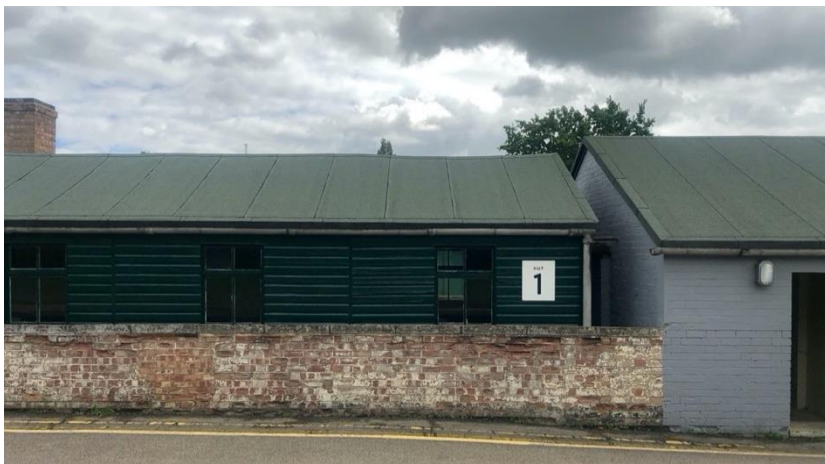
Figure 32 - Bletchley Park hut 1 (Grade II listed)
