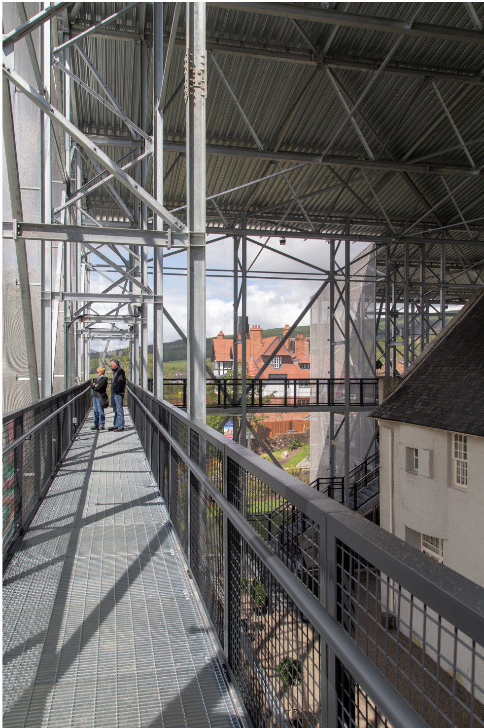
Figure 05. Photographing the Hill House roof from the external walkway.
