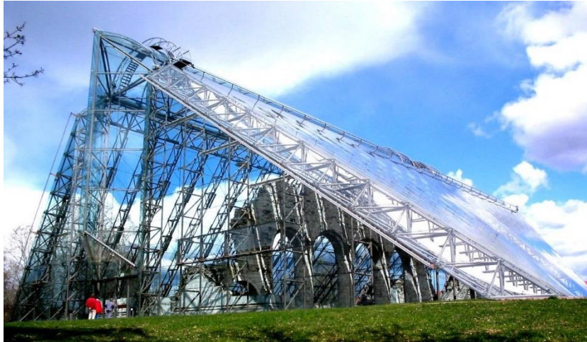
Figure 23 - Old Hamar Cathedral, Norway, complete with protective glass structure
