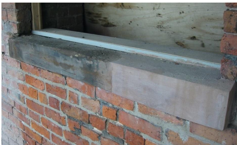
Figure 25 - Isolated sandstone repair at Murrays’ Mills, Manchester. A ‘restored’ sill?
