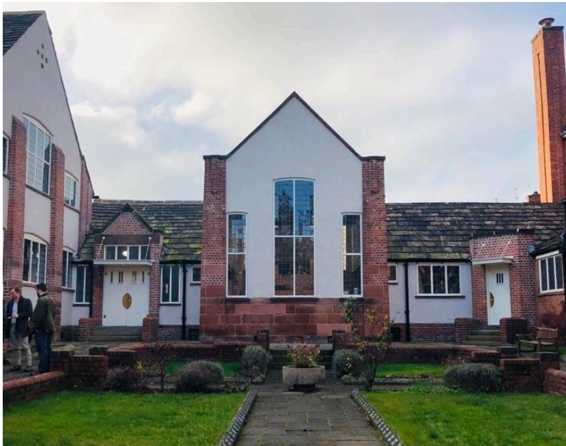
Figure 11 - Long Street Methodist Church and Sunday School (Grade II* listed)
