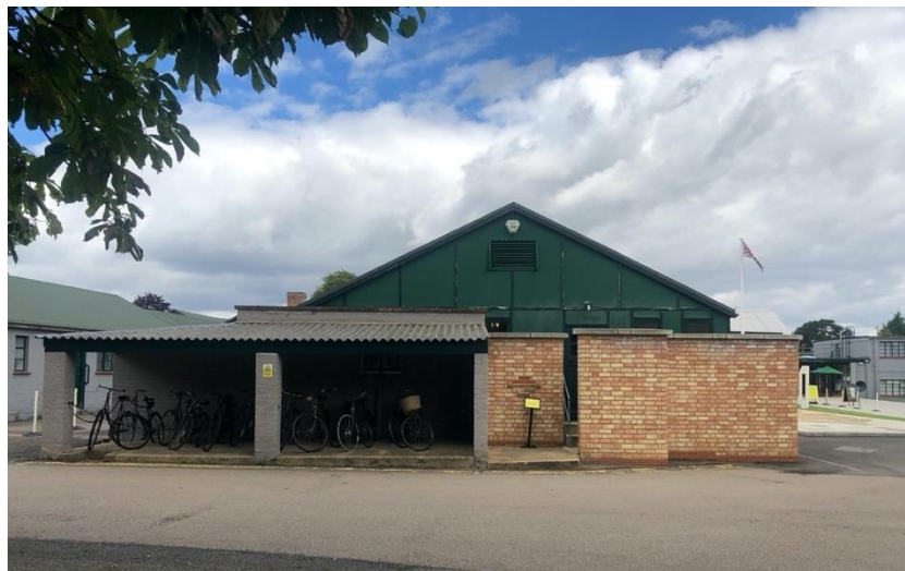
Figure 81 - Hut 8 exterior (with bike shed in front)
