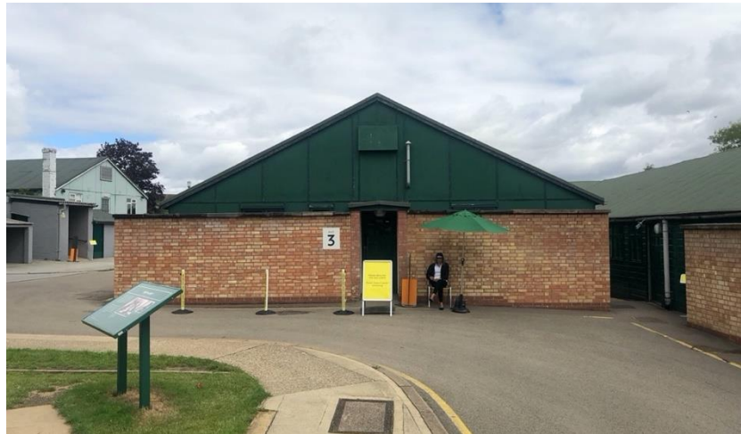
Figure 76 - Hut 3 exterior (behind the reconstructed blast wall)
