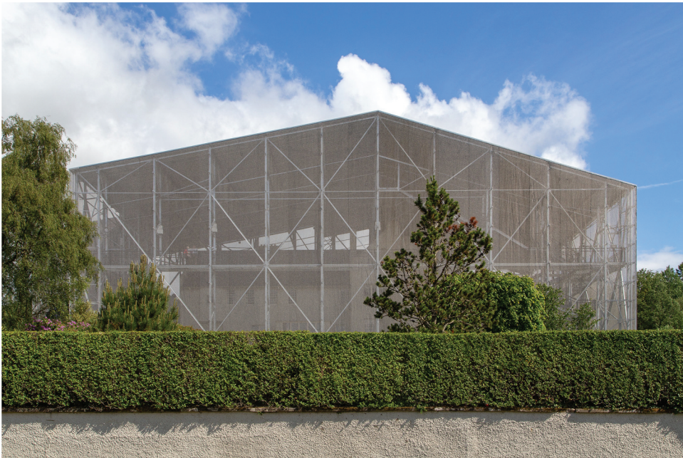
Figure 4. The Hill House encapsulated by the ‘Hill House Box’. Photo: Tom Parnell (CC BY-SA 2.0). Source: https://www.flickr.com/photos/itmpa/48672523318/in/album-72157710676927421/ .
