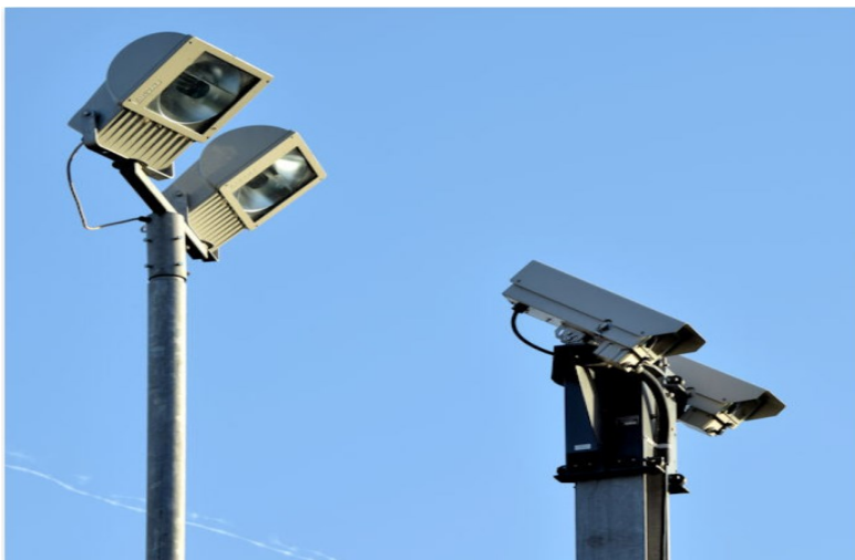
Figure 10A CCTV system installed at a Level Crossing site. Note the flashlights installed along with the CCTV as well to provide enough light for CCTV to operate at low lightning conditions.
