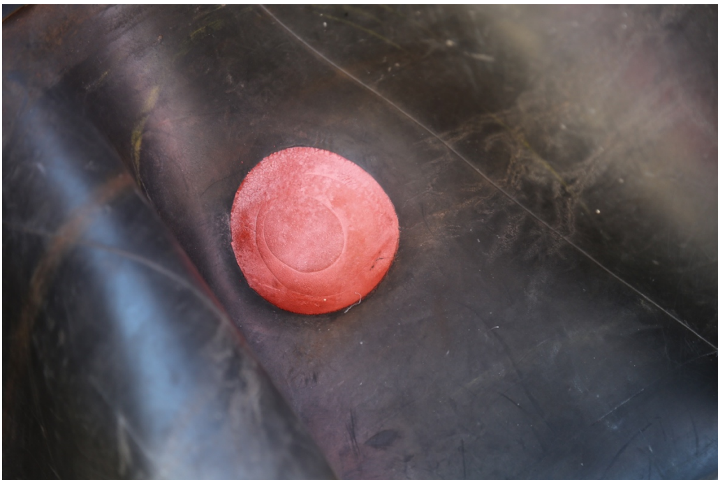
Figure 5 patched tubes detail. 2012
