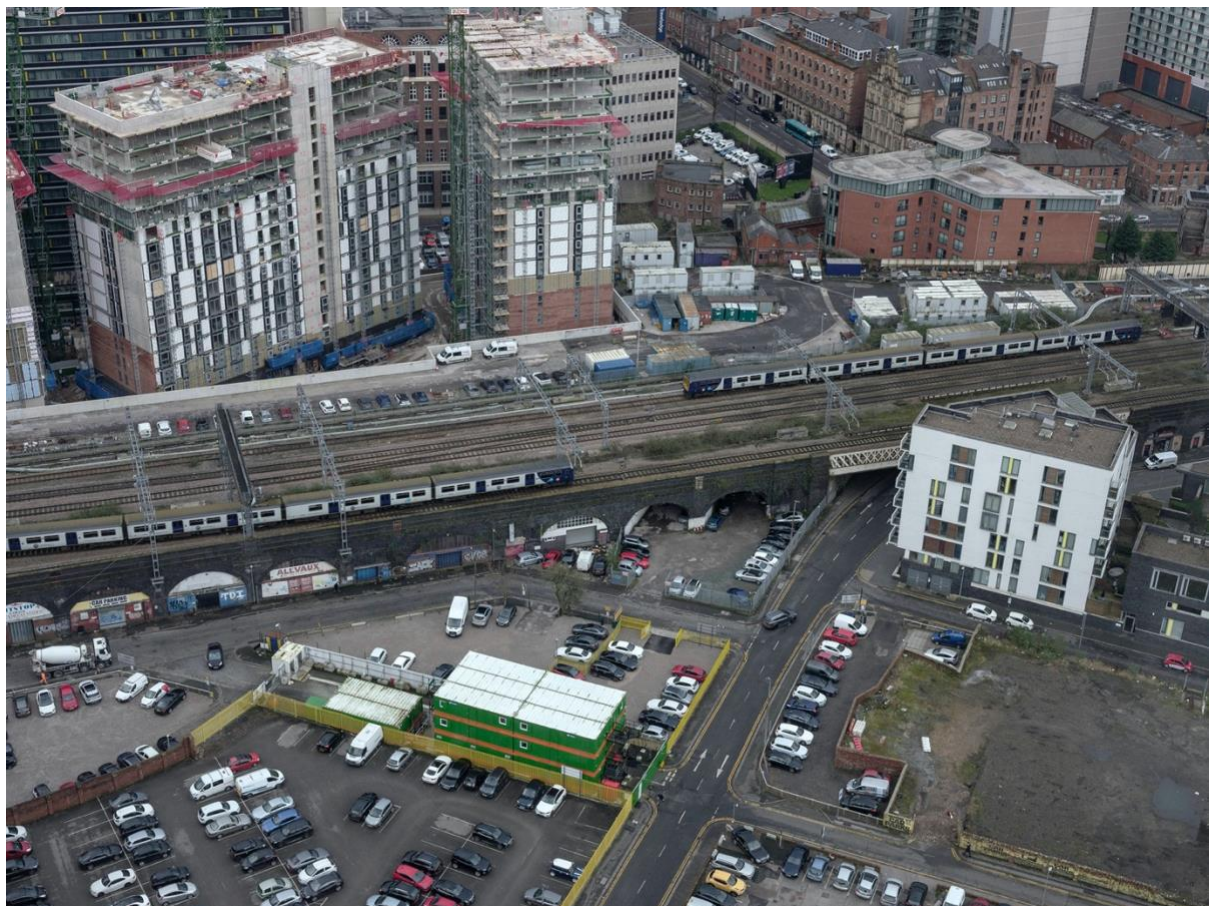
Figure 3: View from Anaconda Cut Apartment, Salford – Image Credit: John van Aitken (2020)
