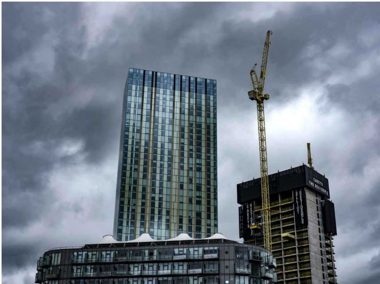
Figure 2: Anaconda Cut, Salford – Image Credit: John van Aitken (2020)
