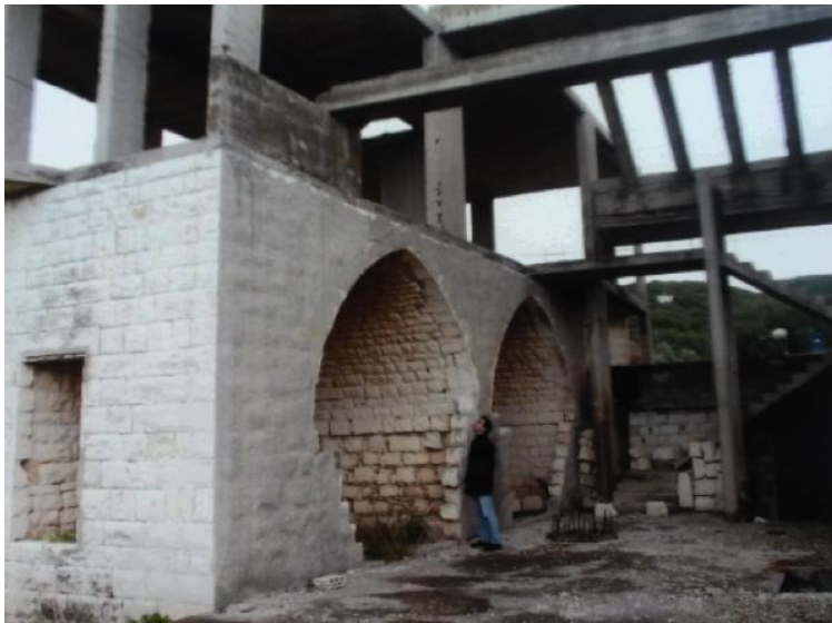
Figure 2 Beginning of the restoration project in 2003
