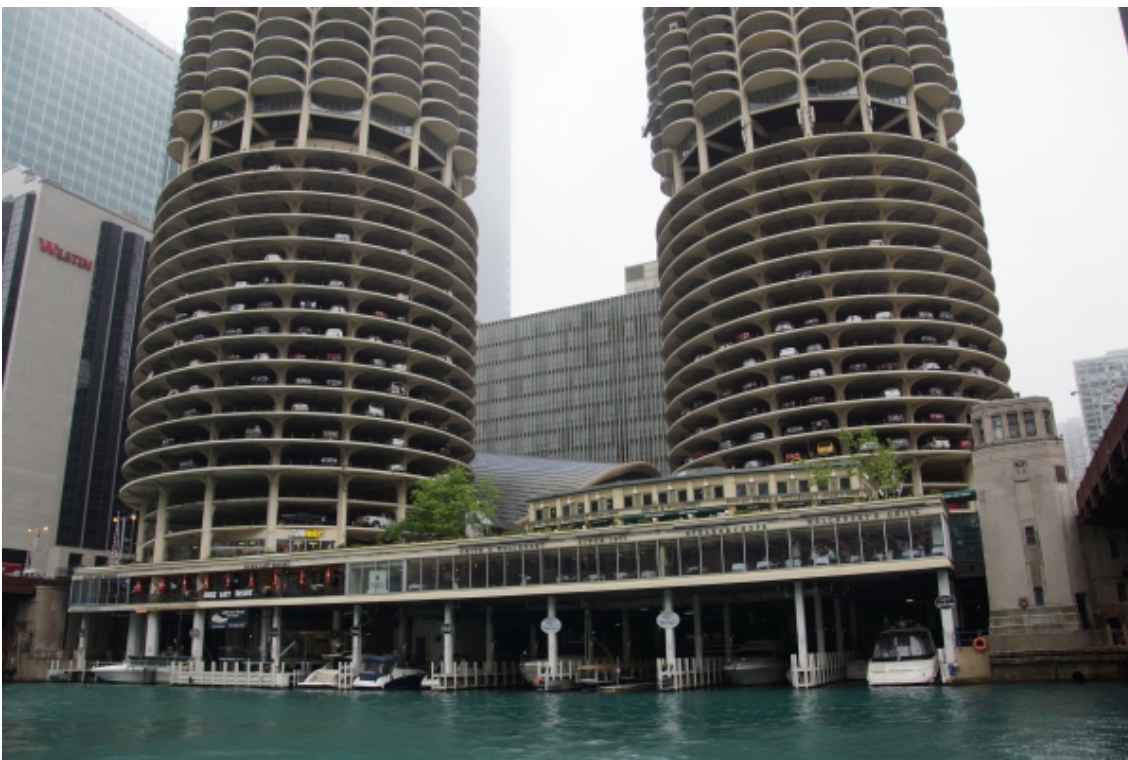
Figure 1.9. Marina City in Chicago is one of the most iconic examples of “carcitecture” where there has been a deliberate attempt to seamlessly integrate the automobile into the design of the building (Source. Nicolas Janberg - structurae.net, 2015).
