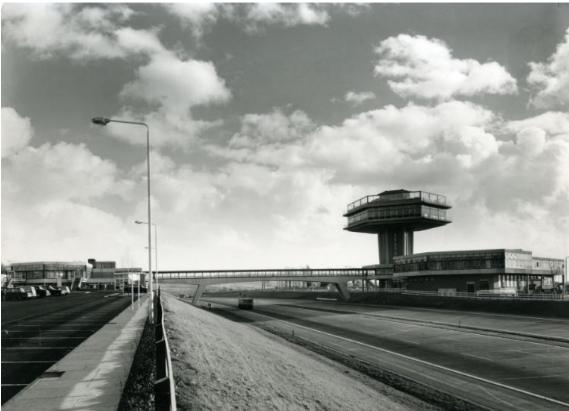
Figure 1.10. The UFO-like structure of Forton Services acts as a landmark against the backdrop of the monotonous motorway network. The platform allows visitors to stop and reconnect with the surrounding landscape (Source: fortonservices.webs.com ).
