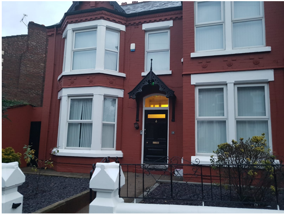
Fig 41. Tom Harrison House in Anfield, Liverpool.
