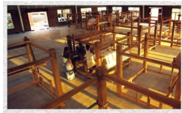
Figure. 4 a. Inside a newly built loom shed at Five P Venture
