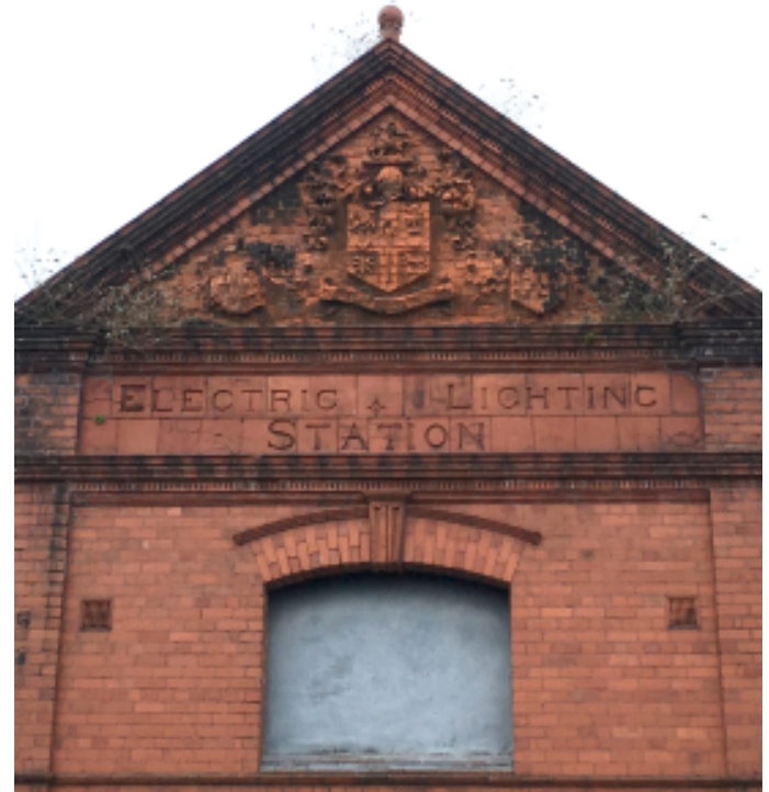
Above: Electric Lighting Station, opposite The Hive. Previous page: Kwong Lee's video installed in Central Library.
