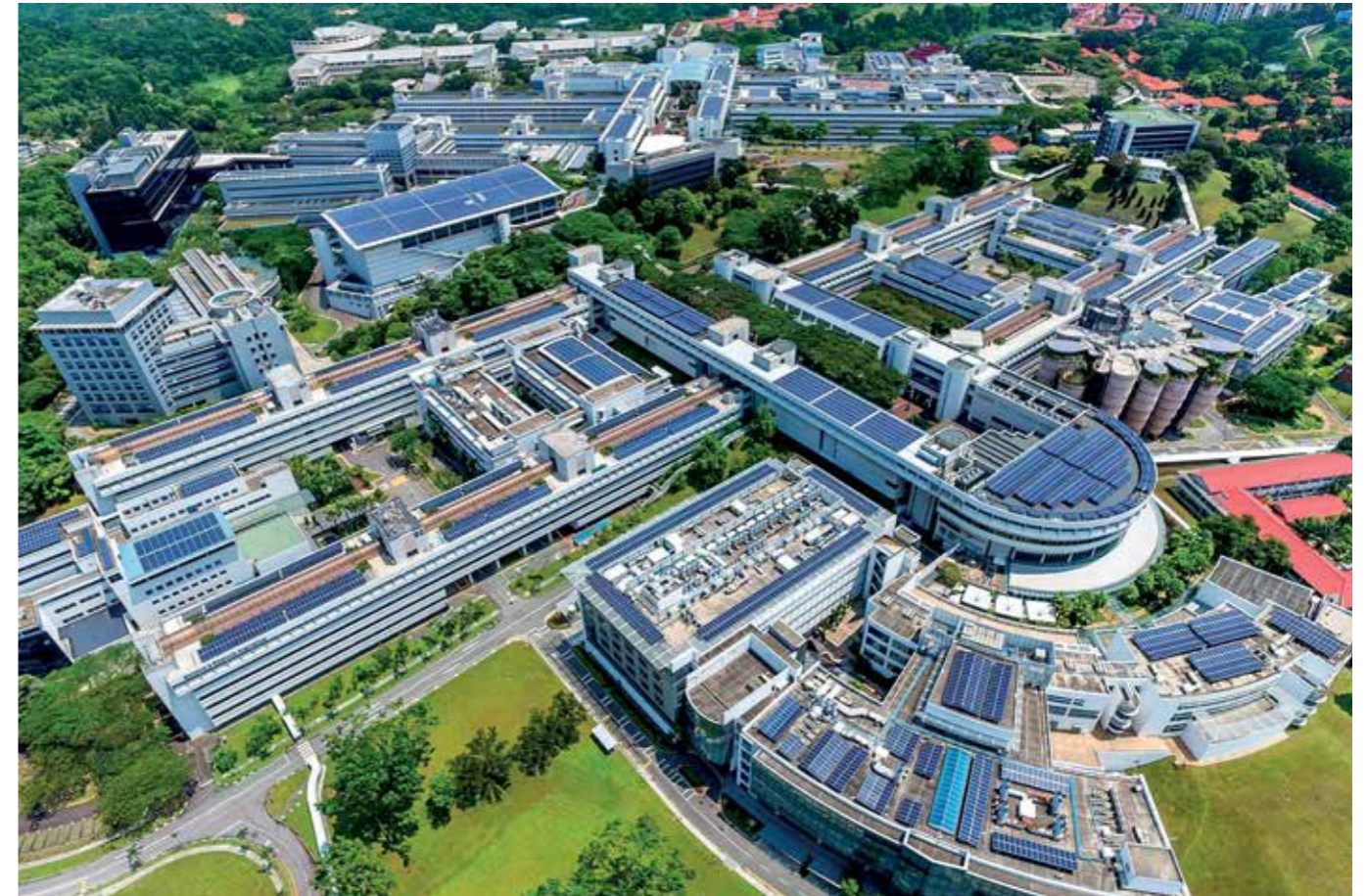
▲ Figure 6. Image of the 5,000 kW rooftop solar photovoltaic installation at NTU Singapore campus (© Nanyang Technological University Singapore).
