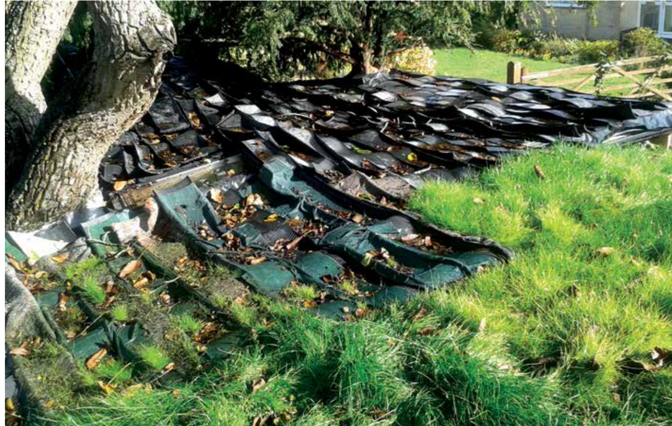
▲ Figure 1. Cut and arranged tyres forming the lattice roof of the Earthhouse (© Christopher Norris).
