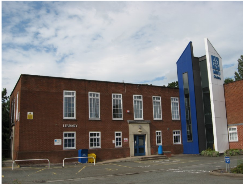
Plate IX: The Crewe campus library of Manchester Metropolitan University showing the library housed in the new library and administration building from the early 1960s. In its last iteration the library service occupied the whole of the building (Photograph courtesy of Crewe Library).
