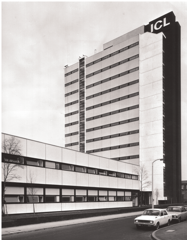
Figure 11 John Seward for Cruickshank & Seward, International Computers Limited Building, West Gorton, England, 1971 (Cruickshank & Seward Archive, Manchester Metropolitan University Special Collections).
