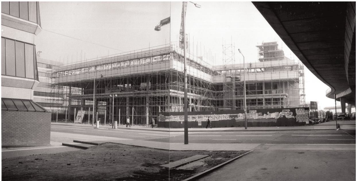
Figure 15 Cruickshank & Seward, National Computing Centre, ca. 1973, construction view with Mancunian Way at right, Municipal College of Technology at left, and BBC North headquarters in the background (Cruickshank & Seward Archive, Manchester Metropolitan University Special Collections).
