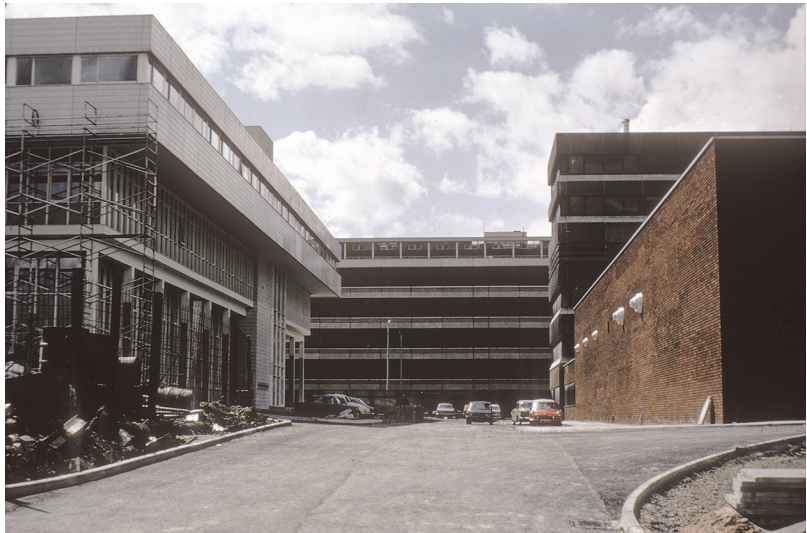
Figure 5 W. B. Heppell, Municipal College of Technology, Manchester, after completion of second phase, 1974, view from across Oxford Road, with National Computing Centre at left and BBC North headquarters at right (ZX-283, Manchester Metropolitan University Special Collections).
