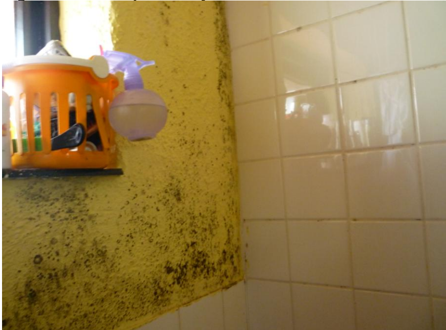
Figure 4.5.4 Damp in utility block
