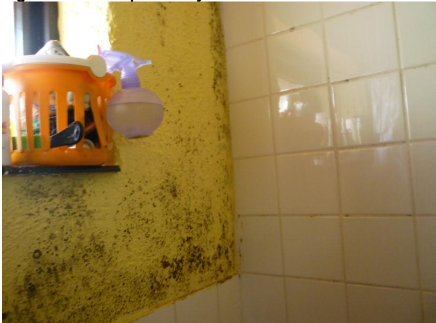
Figure 4.5.4 Damp in utility block
