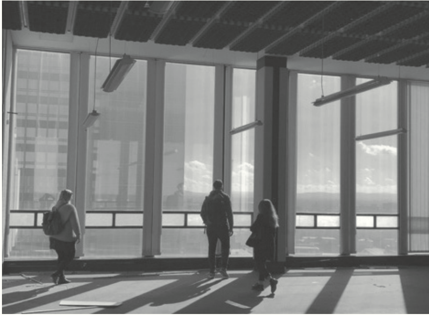
13 th Floor Century House , 2018. Image by Sally Stone.
