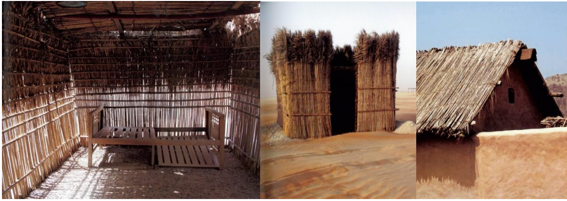
Figure 1.29: Interior and exterior view of a palm leaf transitional shelter and implementation of palm leaf in roofing (Piesik, 2012).
