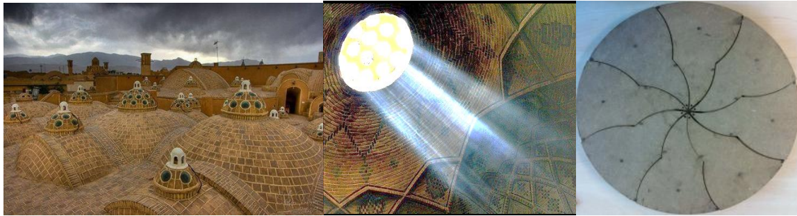
Figure 4.21: Low-tech traditional natural lighting through roof windows in Soltan Ahmad Bath, Kerman, Iran (Left and middle) (Ref. http://deeparternature.blogspot.co.uk/ ), designed erectable window for emergency shelters (Right) (By author)
