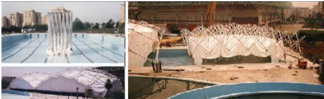
Figure 5.8: Deployable cover for a swimming pool in Seville designed by Escrig and Sanchez. Image Credit Performance SL (De Temmerman, 2007).
