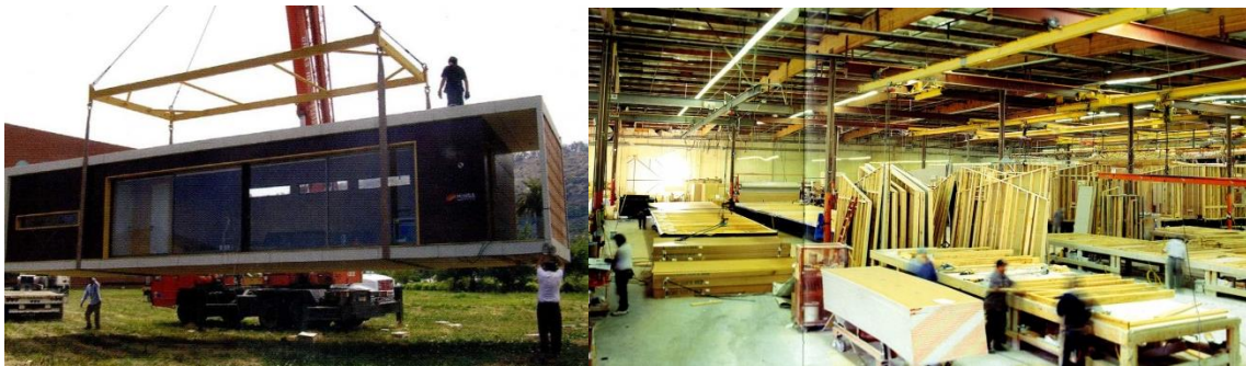
Figure 1.17: Transitional shelter, manufacturing and assembling in factory Credit image: Alejandro Dumay (Arieff and Burkhart, 2003).
