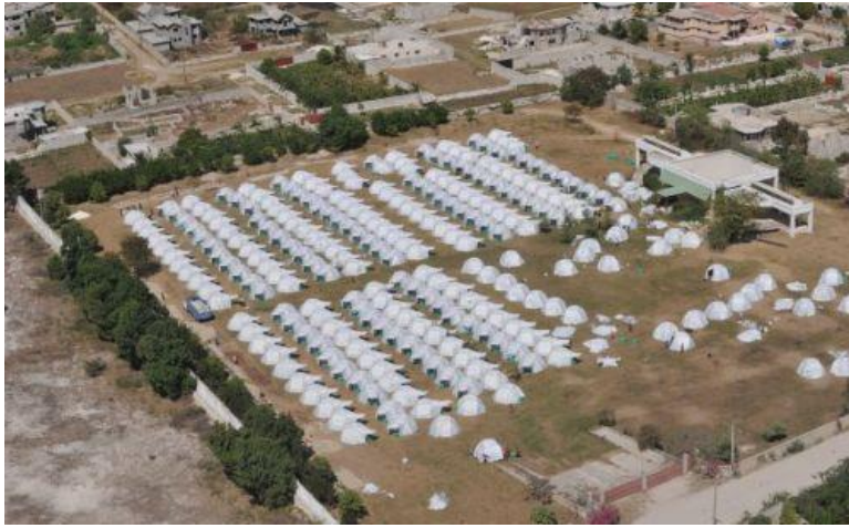
Figure 1.13: Haiti as a poor country, predicted a crisis point for emergency sheltering, a school during the post-earthquake period.
