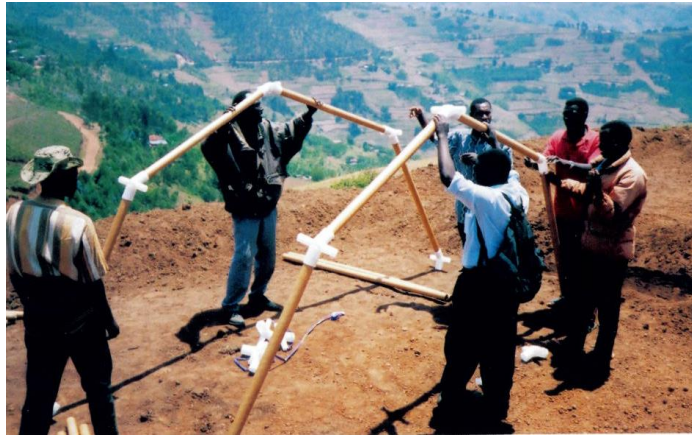
Figure 6.16: A paper tube tent designed by Shigeru Ban (McQuaid, 2003).
