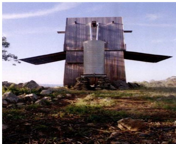
Figure 1.19: A transitional shelter made from corrugated metal sheets (Arieff and Burkhart, 2003)
