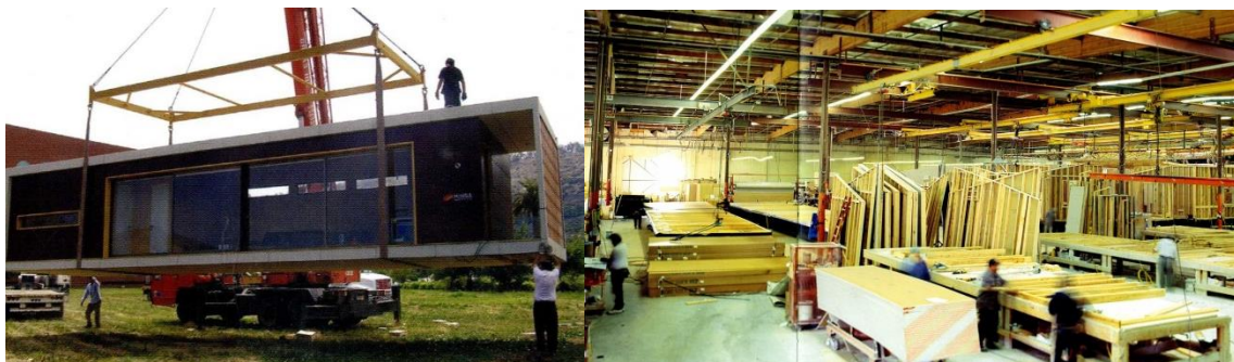
Figure 1.17: Transitional shelter, manufacturing and assembling in factory Credit image: Alejandro Dumay (Arieff and Burkhardt, 2003).
