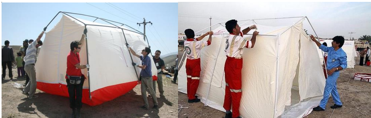
Figure 4.13: Iranian Red Crescent erecting emergency shelters inside the camps (Ref: Mojepishro.net Image Credit: Saeedi, Access date:25/06/2015)
