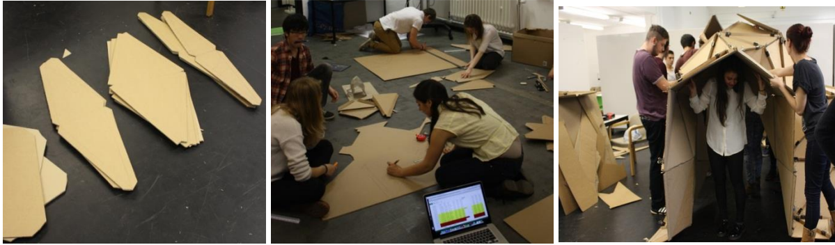
Figure 6.12: Prototyping emergency shelters by un-skilled volunteers aged between 17 – 25 in University. Prototyping includes cutting and assembling the panels. 26 th and 27 th Nov 2013.
