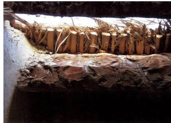
Figure 1.27: Example of implementation of palm-leaf for roofing in abandoned houses.
