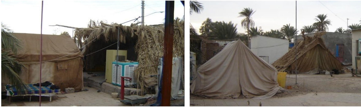
Figure 6.9: Application of palm leaves as a local material in Bam during emergency sheltering (By author).
