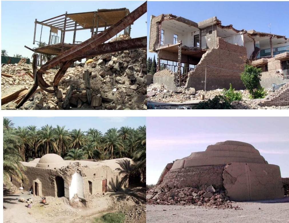
Figure 1.10: Earthquake damages to contemporary (top) and traditional building in Bam (down) (Ref: http://www.earth-auroville.com ).
