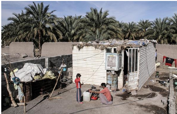
Figure 4.17: Condition of transitional shelters a decade after Bam earthquake (Ref: ISNA News Agency, photo credit :Rahim Baniasad Azad)
