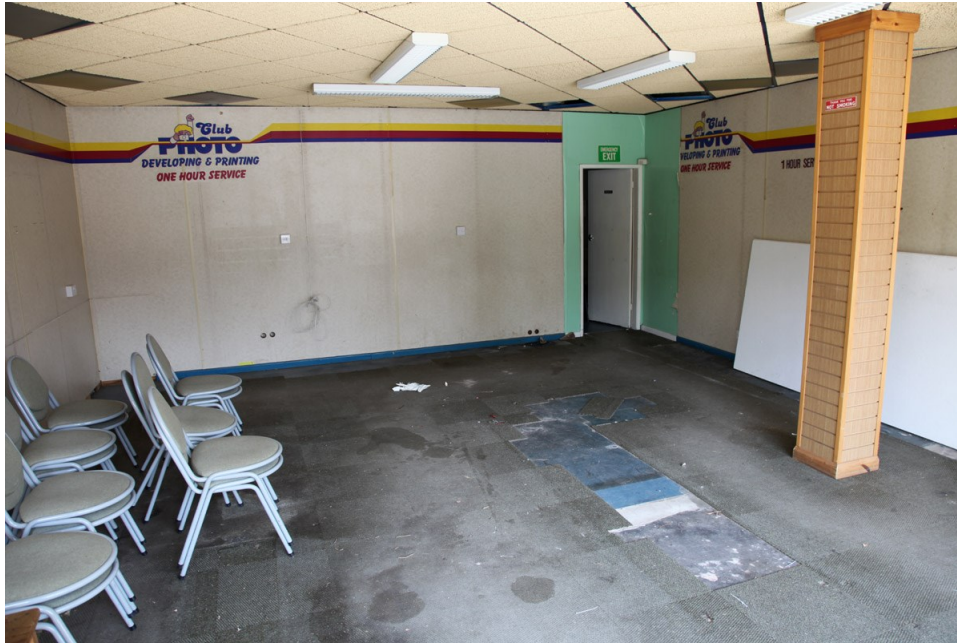
Fig 24 Before: The gallery space as an empty shop
