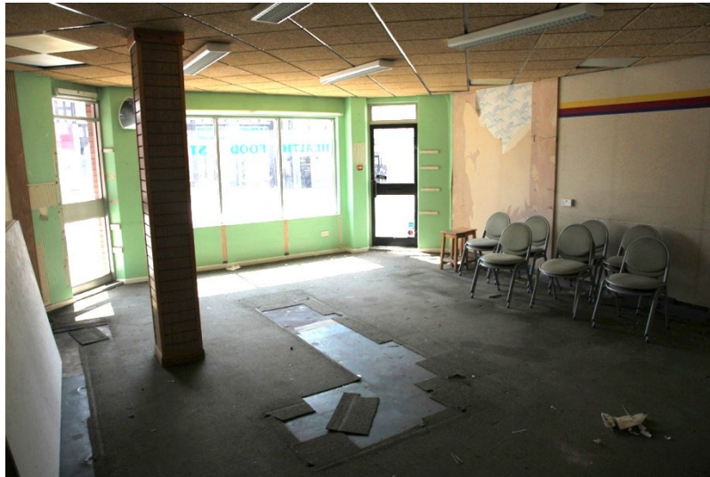
Fig. 22 The former health food shop at 93 Brunner Court before we renovated the building into a second VAC Gallery with lots of volunteer support. Image Alan Carr
